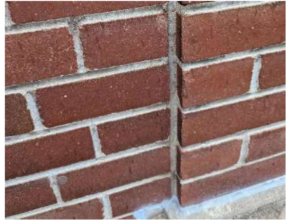
Fig 12: Typical continuous vertical joint at brick pier
