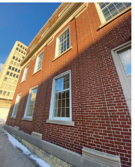
Figure 22. North portion of west facade to be removed.
