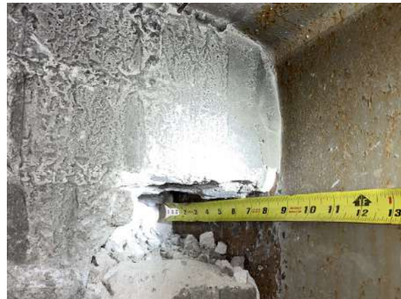
Fig 4: Typical beam bearing length on exterior wall
