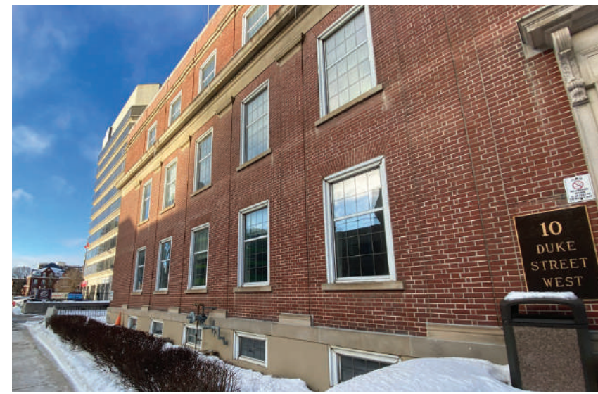
Figure 2. Southwest (left hand side) of Duke St. facade to be retained.
