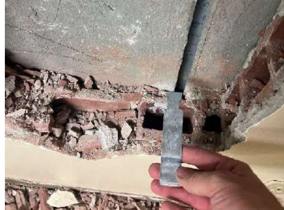
Fig 6: Looking down at opening, dovetail anchor
