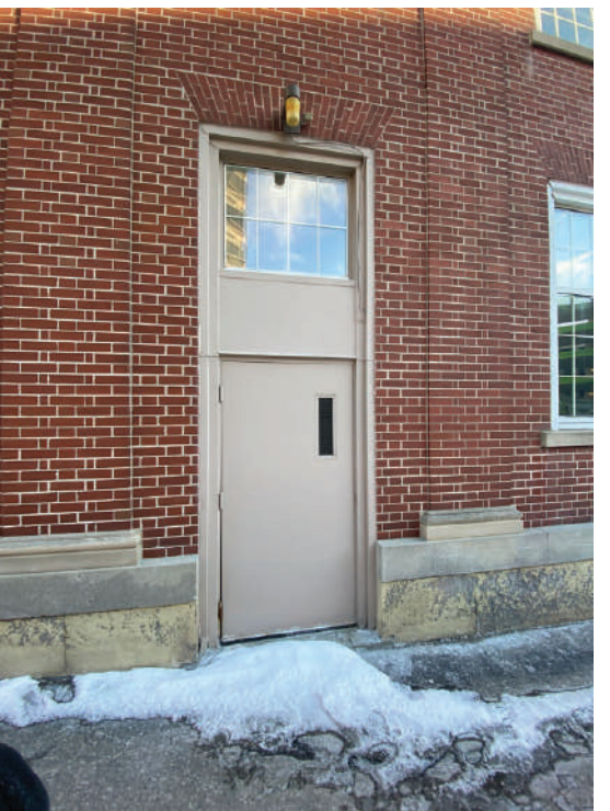
Figure 30. West facade to be retained up to end of this bay.
