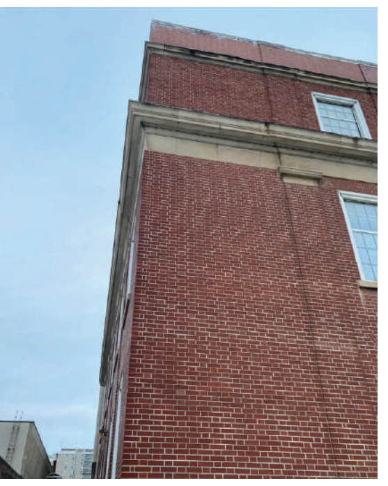
Figure 11. Southwest corner of Duke St facade (left corner)
