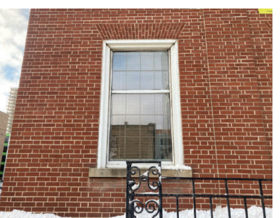
Figure 27. Wrought iron fence at grade on southeast facade.
