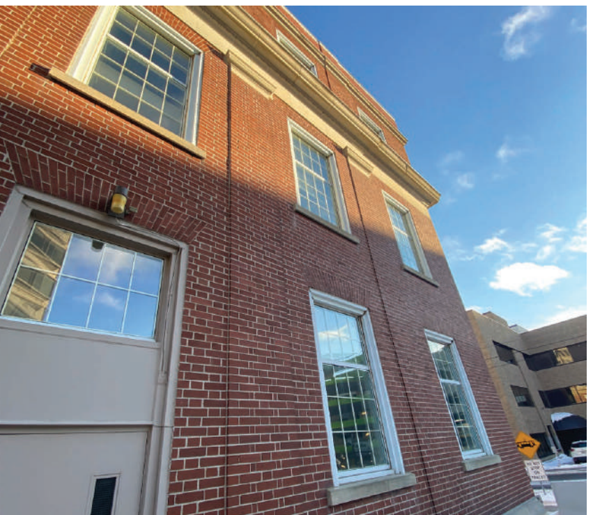
Figure 29. Southern portion of west facade to be retained.
