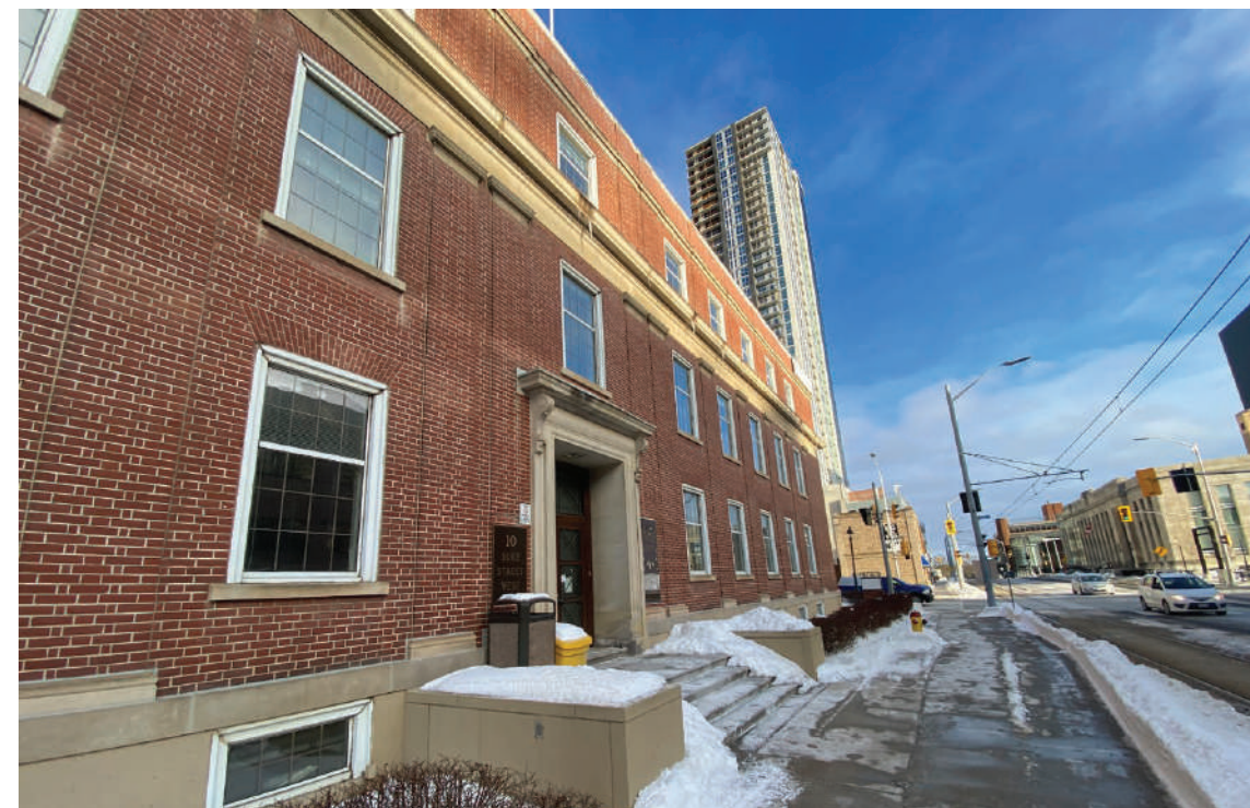
Figure 12. View along Duke St. facade towards Queen St (southwest to southeast).
