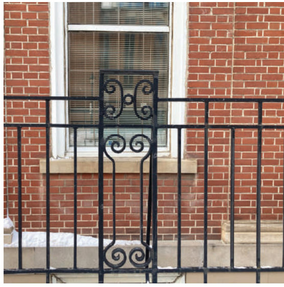
Figure 21. Ornate wrought iron fence at east facade
