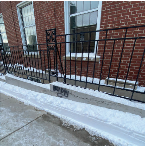
Figure 23. Retaining wall at grade change along Queen St.
