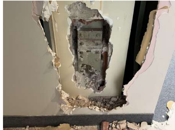
Fig 2: Typical column splice, above 2 nd floor
