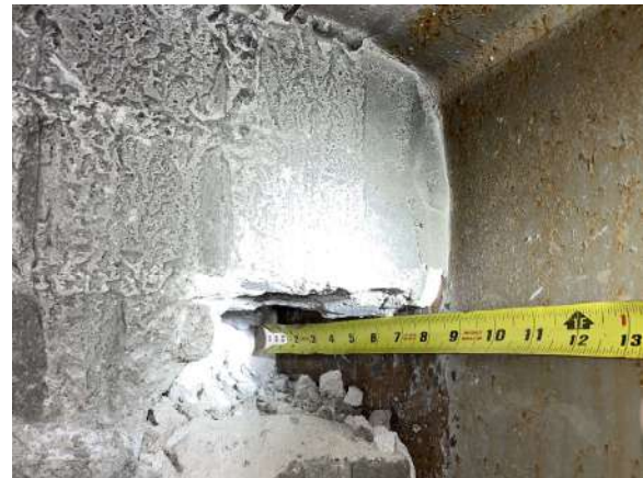
Fig 4: Typical beam bearing length on exterior wall
