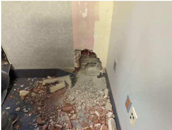
Fig 9: Removals at slab level, S wall, above 2 nd floor
