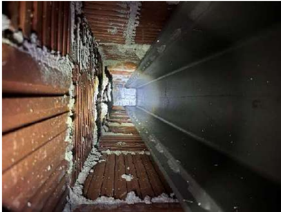
Fig 1: Looking up a column enclosure, from G floor to 2 nd
