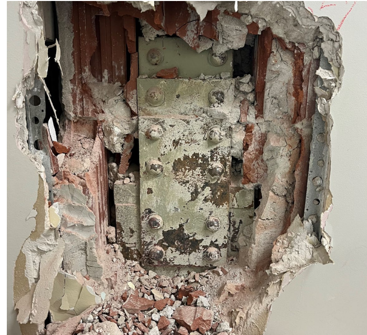
Interior Column Splice
