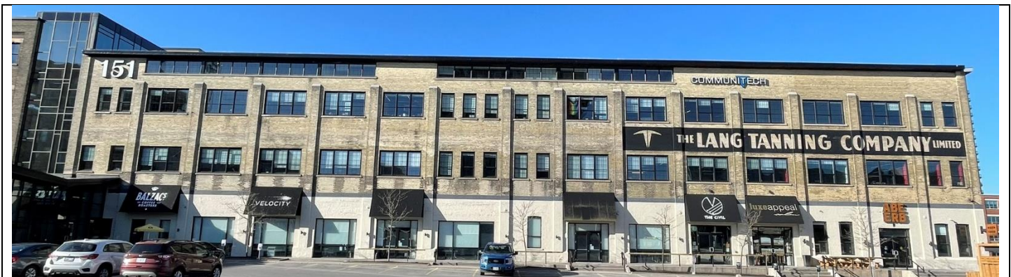
Front Elevation (North Façade) –Former Beam/Storage House of the Lang Tanning Co.
