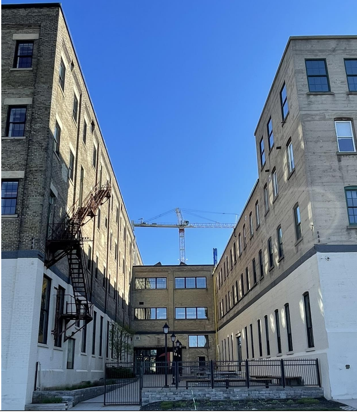
Rear Elevation (South Façade) – New Courtyard
