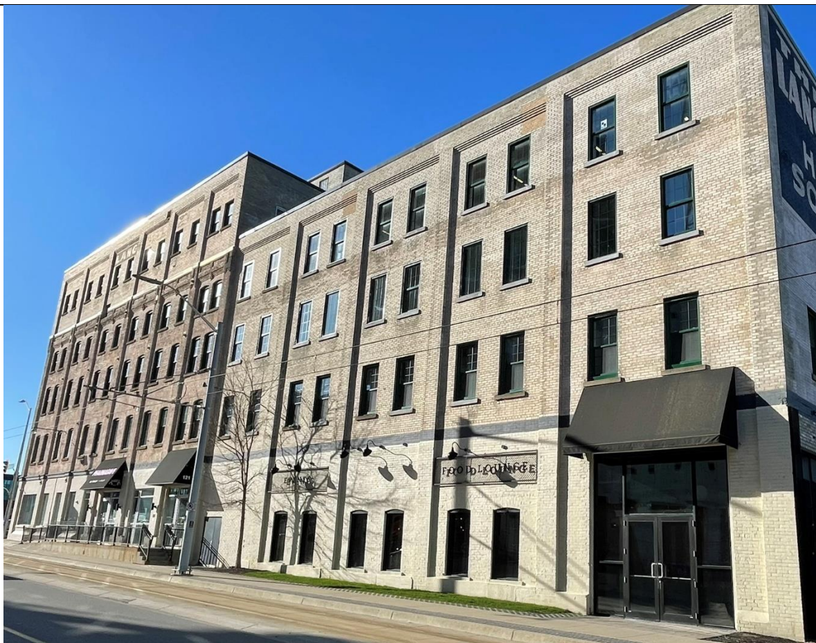
Front Elevation (North Façade) – Former Administration and Tan Yard Buildings of the Lang Tanning Co.
