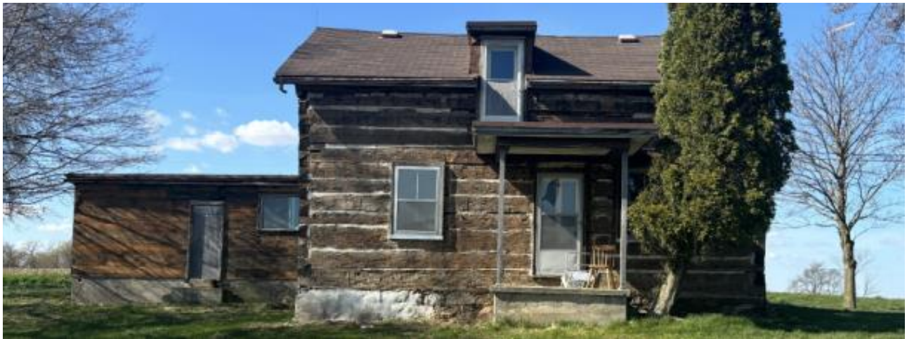
Figure 2.0: Front Elevation of Log House (South Elevation) with one-storey building addition on the left
