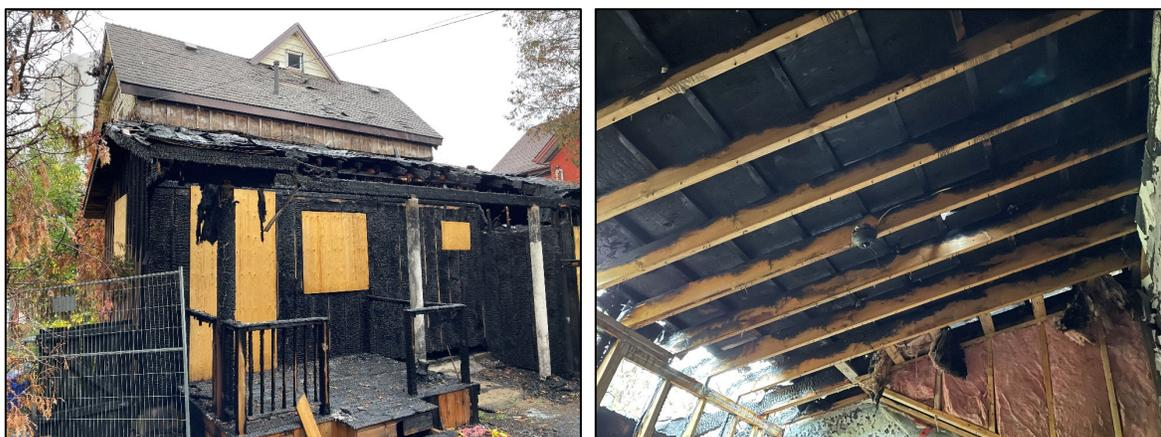
The roof framing above the garage addition was concealed at the time of our review; however, it appears that this roof framing was likely also at least locally damaged by the fire.
