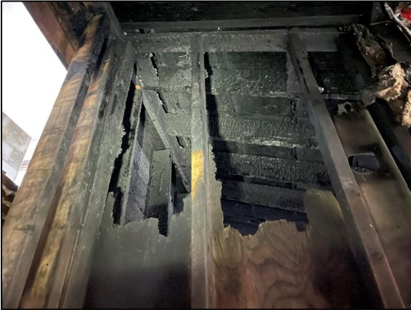
The fire also damaged the majority of the rear exterior wall of the first-floor bedroom and bathroom within the addition. The full extent of damage to the wall is subject to confirmation; however, it appears that the exterior edge at the top of the wall studs were damaged along the majority of the rear wall.
