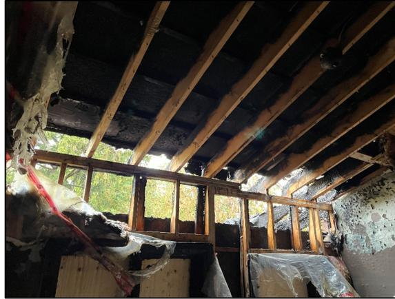
The fire damaged the rear exterior deck as well as the rear ends of the first-floor joists of the addition. Where checked, the floor does not appear to have included a rim joist along the rear exterior wall, allowing the fire to enter the crawl space. The full extent of damage to the currently concealed floor joists is subject to confirmation and will likely require the removal of the floor sheathing.
