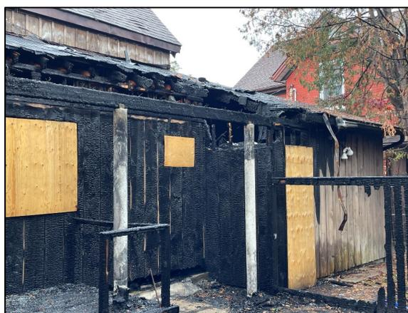
Fire damage to the roof extended up and damaged the top of the interior loadbearing wall where the roof of the rear addition meets the original building above the laundry room. This wall appears to have been constructed on the exterior side of the original brick masonry and is assumed to provide loadbearing support for the roof of the addition. It is subject to confirmation following the removal of interior finishes if the adjacent wall of the original building was also damaged.
