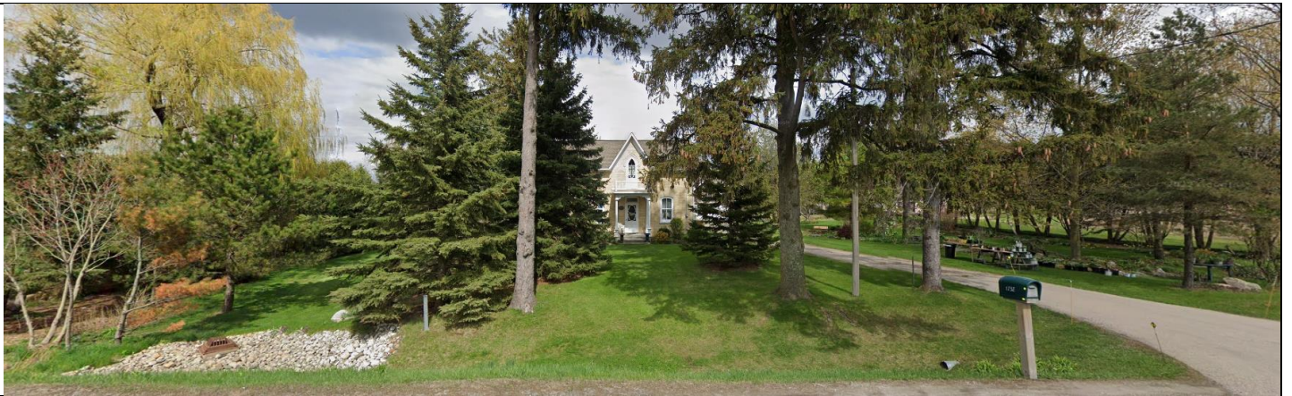
Wide Angle View of the Frontage of the Property, including the Front Elevation (West Façade) of the Farmhouse – 1738 Trussler Road
