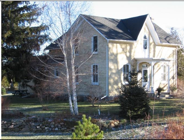
Front and Side Elevation (West and North Façade) – 1738 Trussler Road
