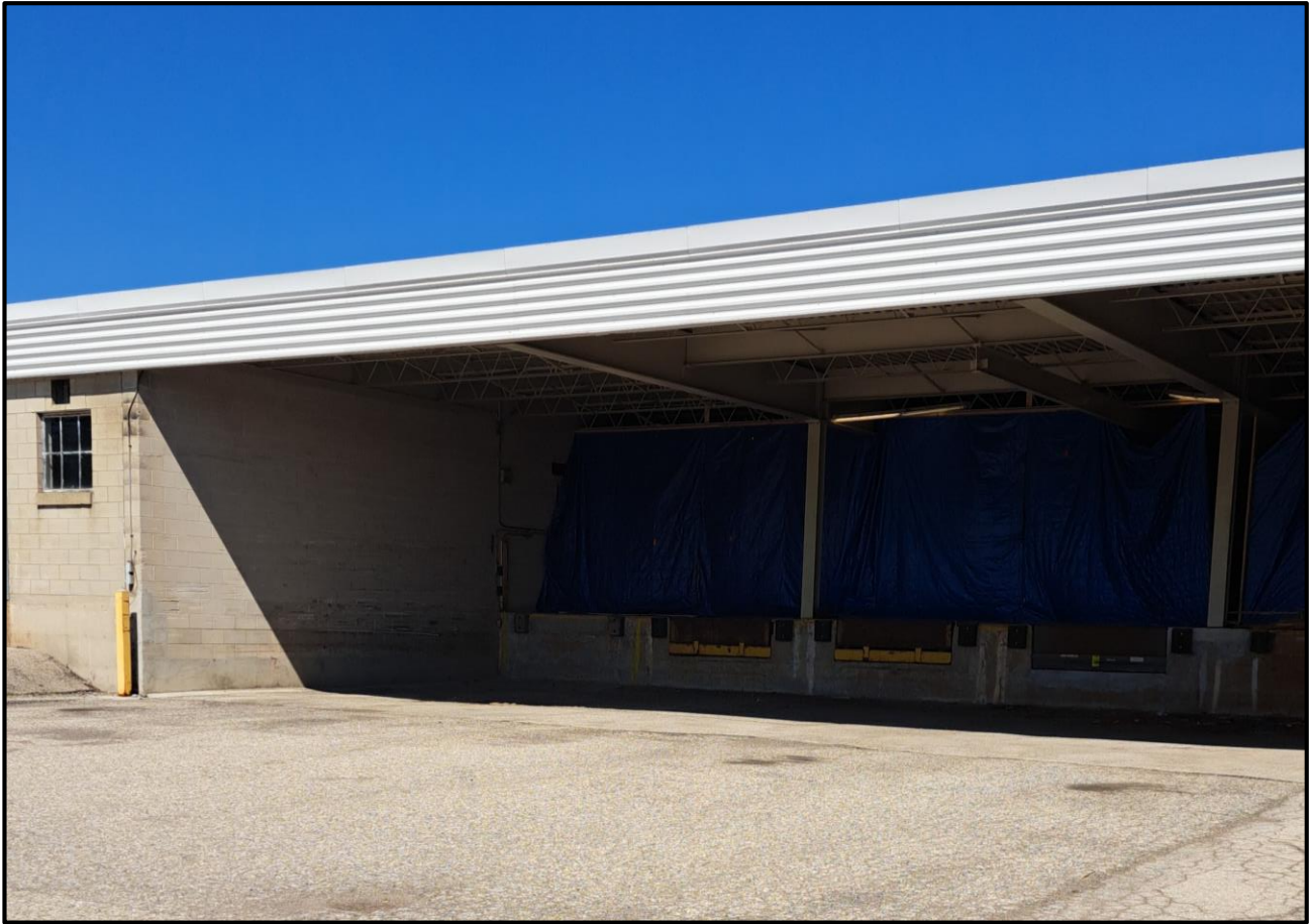
Figure 5: A photo of the building side that will be closed.
