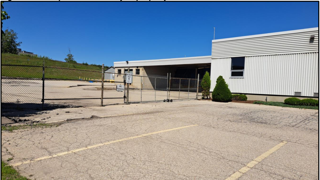
Figure 4: West photo of the subject property showing the existing loading area.
