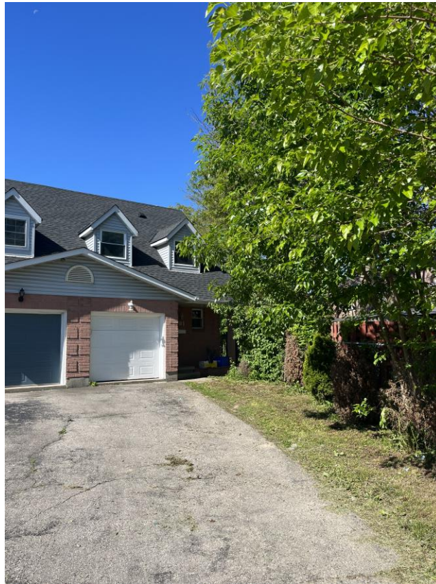
Figure 4 - View of 101 Breckenridge Drive from the Street.
