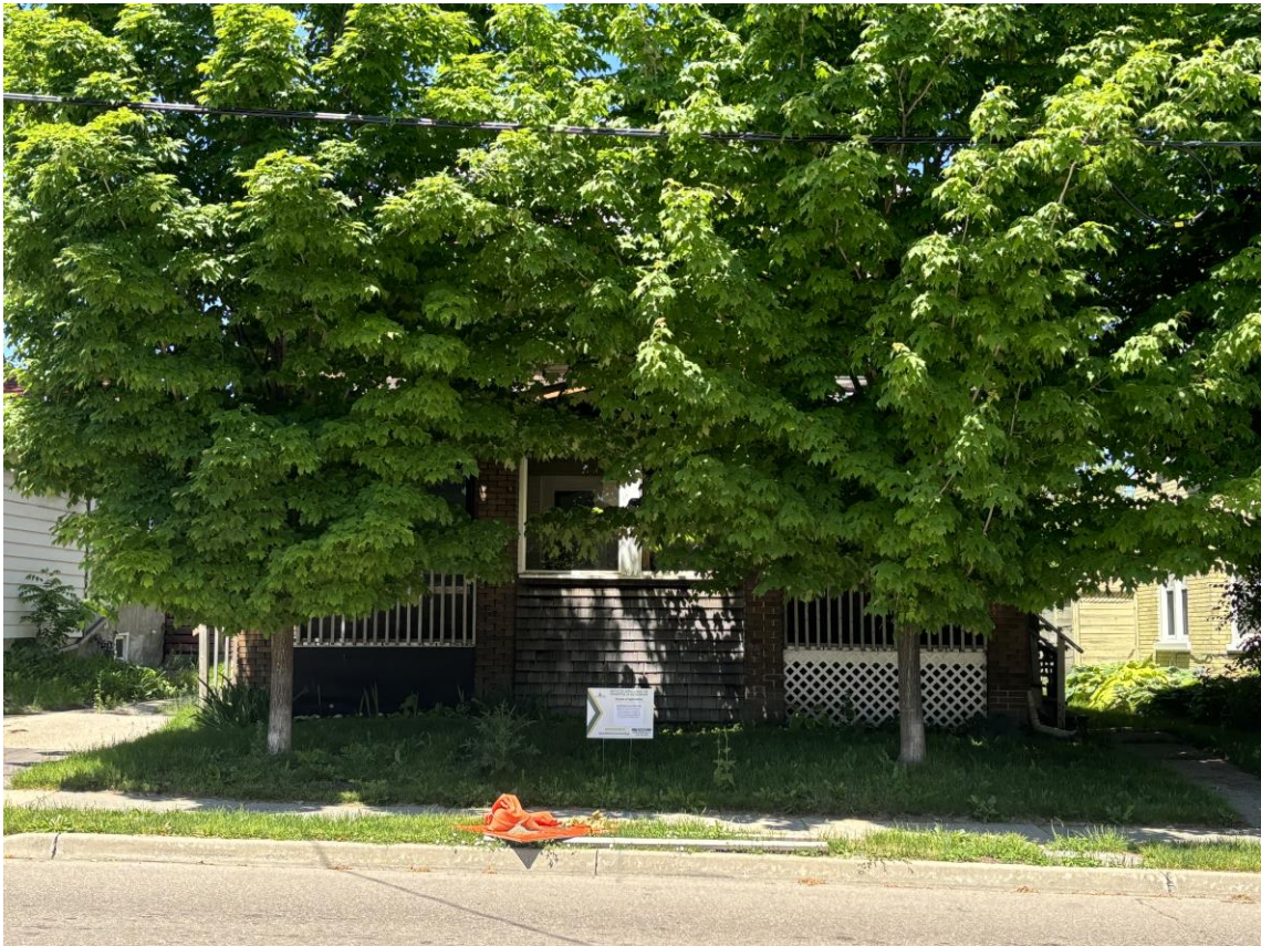
Figure 5 - View 174 Wellington Street North from the street.
