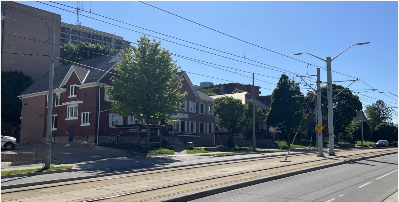
Figure 3: Existing site conditions of 47-63 Charles Street East and 75 Charles Street East.
