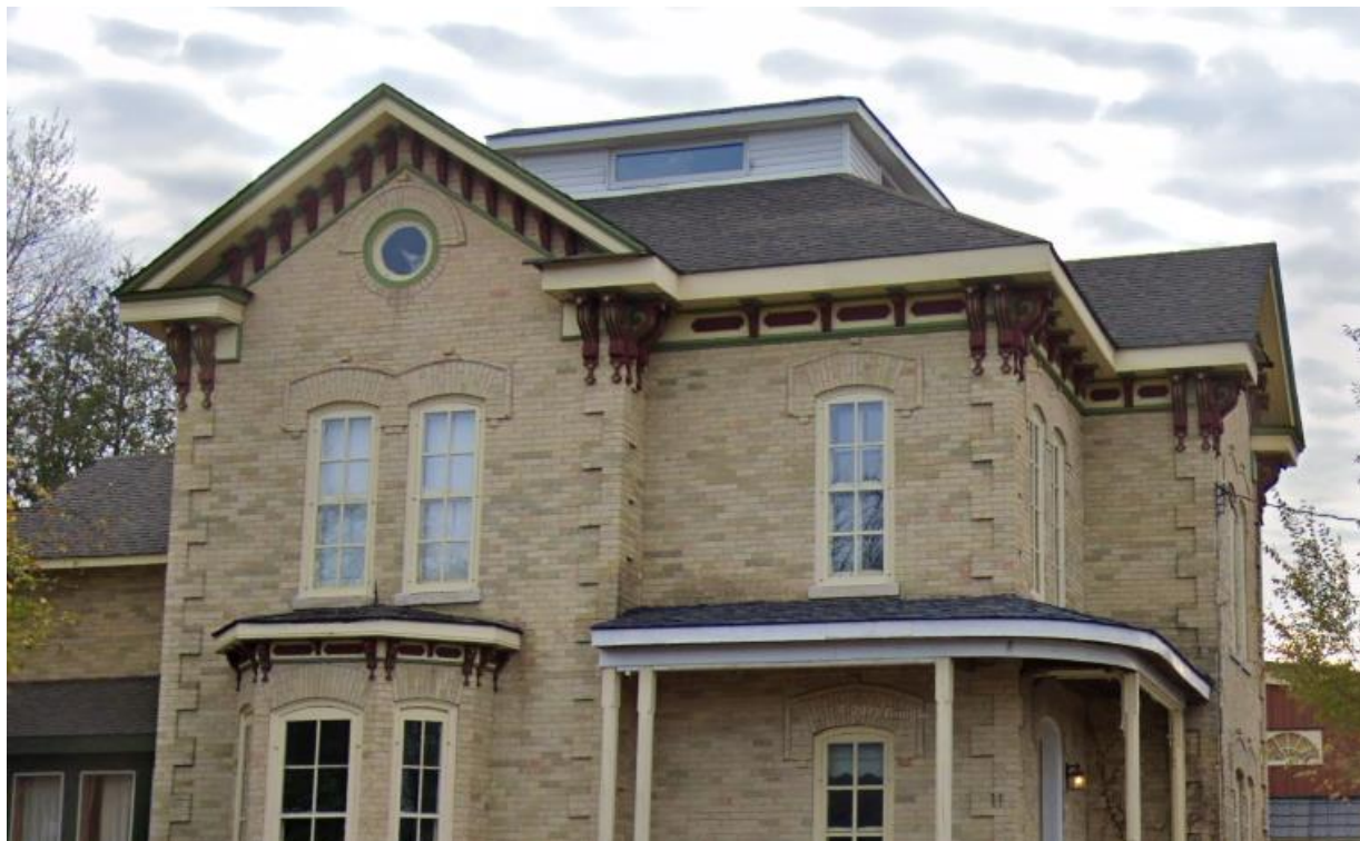
Figure 3.0: Detailing of truncated hip roof with cross gables; central hip roof that leads to the clerestory windows; moulded fascia, plain cornice, and panelled frieze with paired brackets; projecting centre bay on west elevation with bay window; double (suspected) yellow brick construction; corner brick quoins; segmentally hung wood windows with decorative hood crowns, and stone sills. (Google Streetview, 2020)
