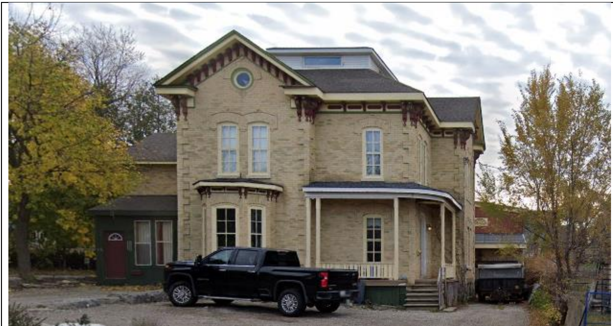
Front Elevation (West Façade) (originally a side elevation) (Google Streetview, 2020)
