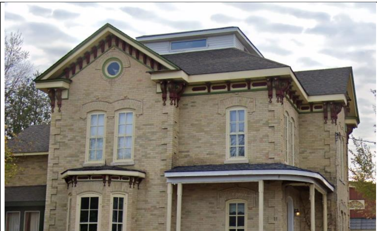
Detailing of truncated hip roof with cross gables; central hip roof that leads to the clerestory windows; moulded fascia, plain cornice, and panelled frieze with paired brackets; projecting centre bay on west elevation with bay window; double (suspected) yellow brick construction; corner brick quoins; segmentally hung wood windows with decorative hood crowns, and stone sills. (Google Streetview, 2020)
