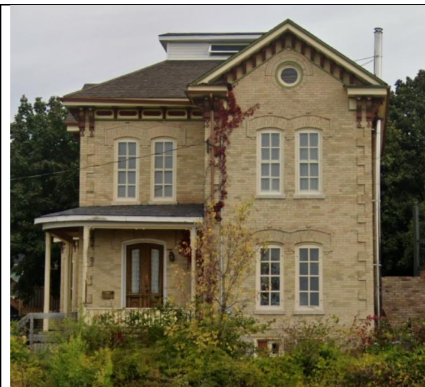
Side Elevation (South Façade) (originally the front elevation off of King Street East) (Google Streetview, 2023)
