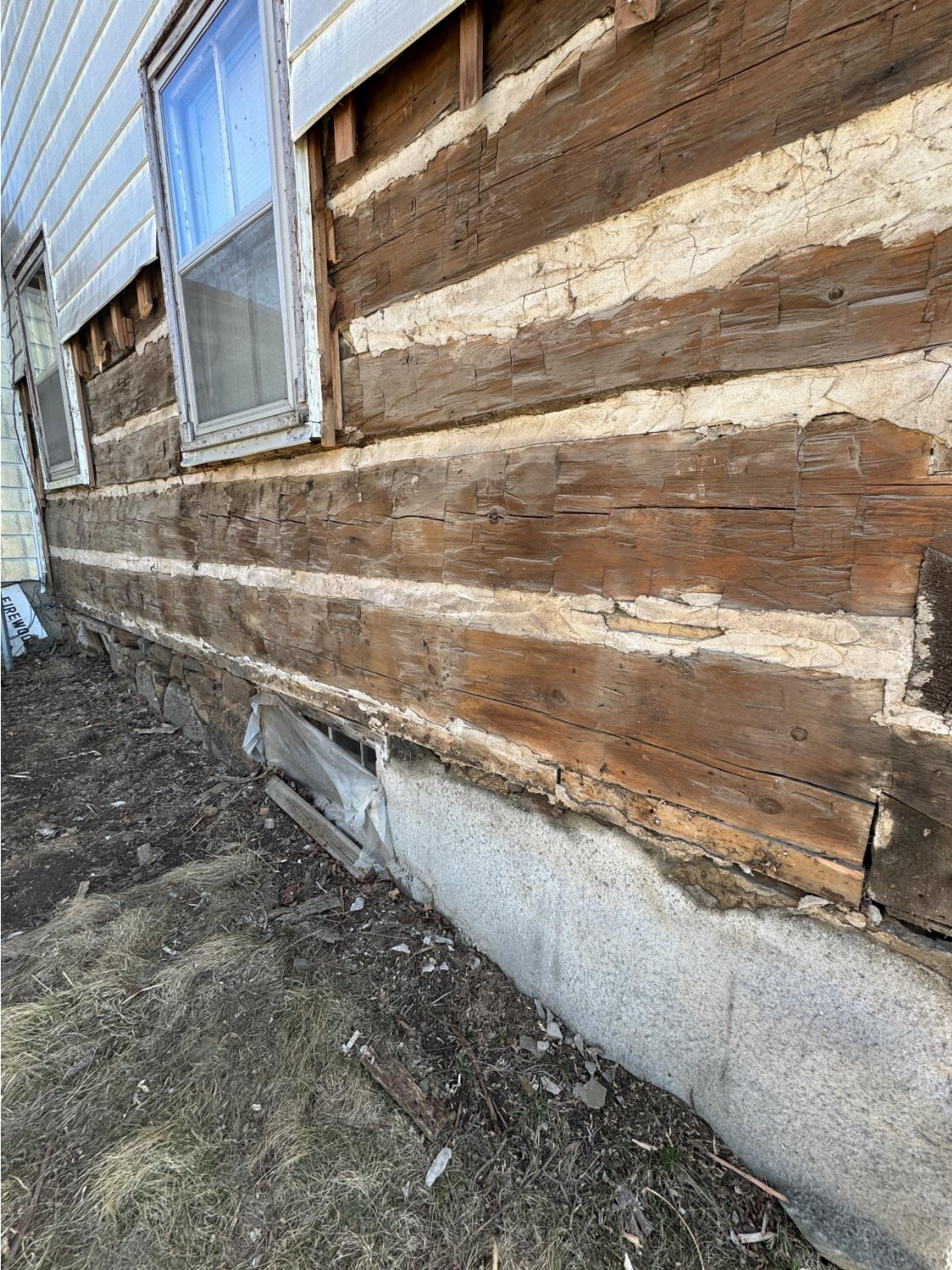
Photo #8: West elevation, partially parged foundation, exposed wall with chinking
