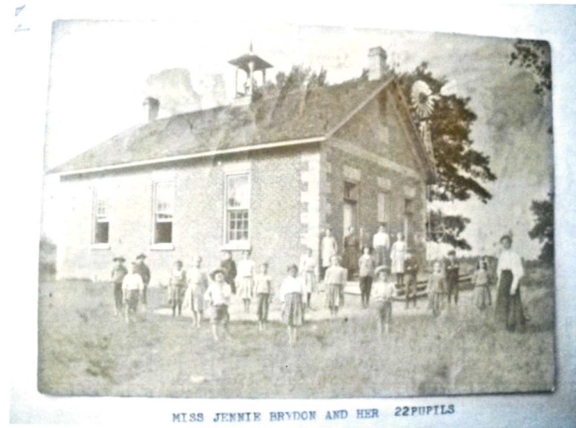
Figure 40: Photograph from the Tweedsmuir History Book of the Plains School House prior to any alterations
