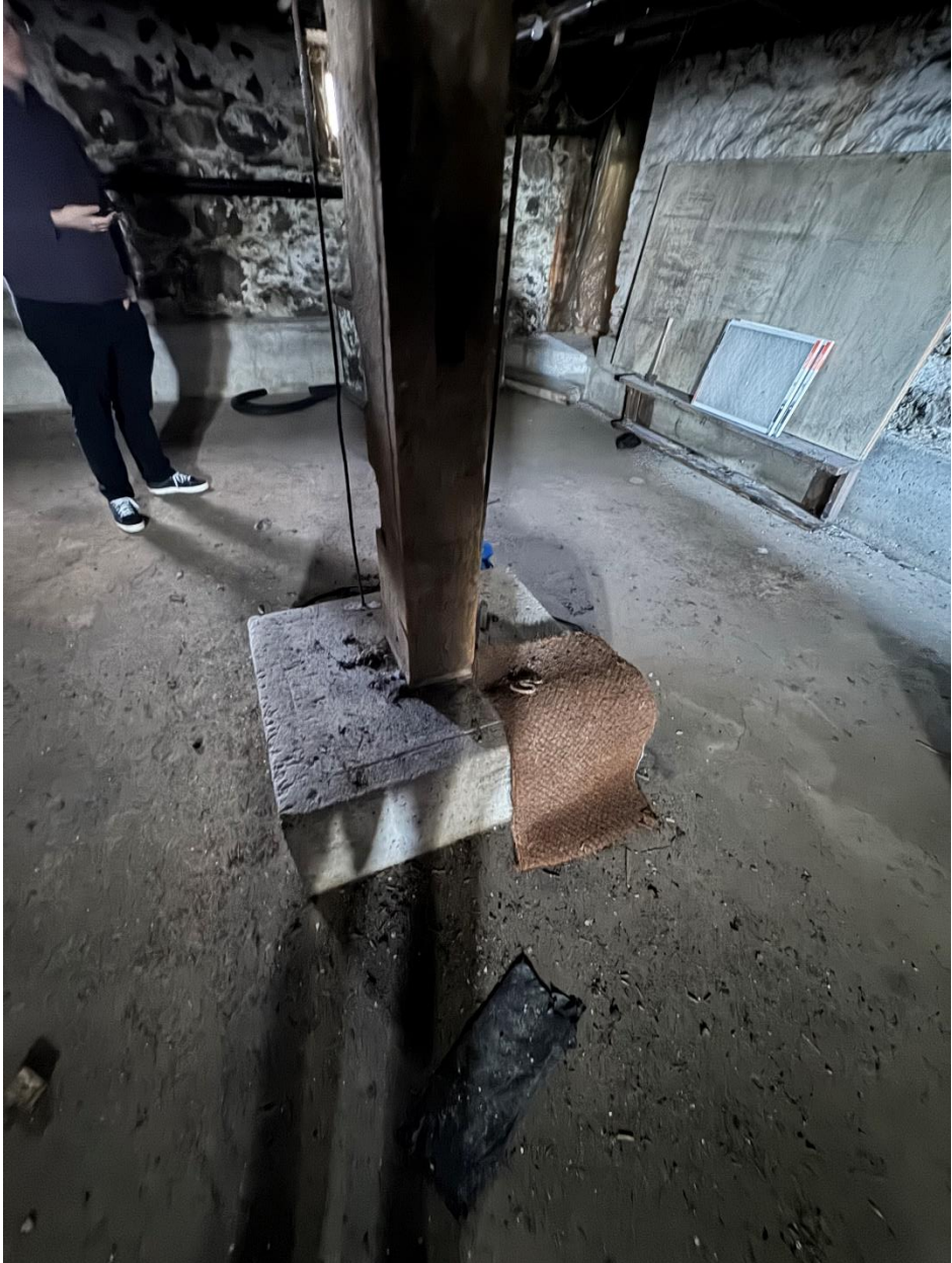
Photo #15: Central column on pad footing
