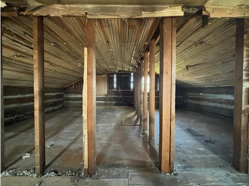
Photo #17: Roof framing finishes removed.
