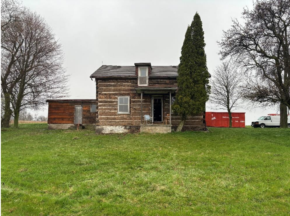
Photo #3: South Elevation (exterior finishes removed)
