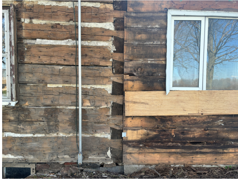
EAST SIDE JUNCTION OF LOG STRUCTURE TO 1- STOREY ADDITION
