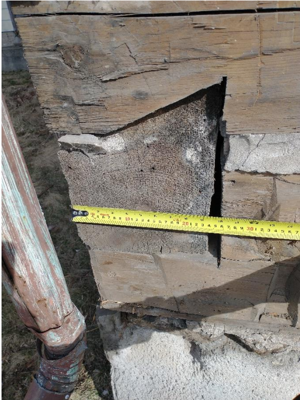
Photo #9: Corner log measurement
