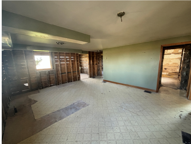
KITCHEN LOOKING SOUTHEAST
