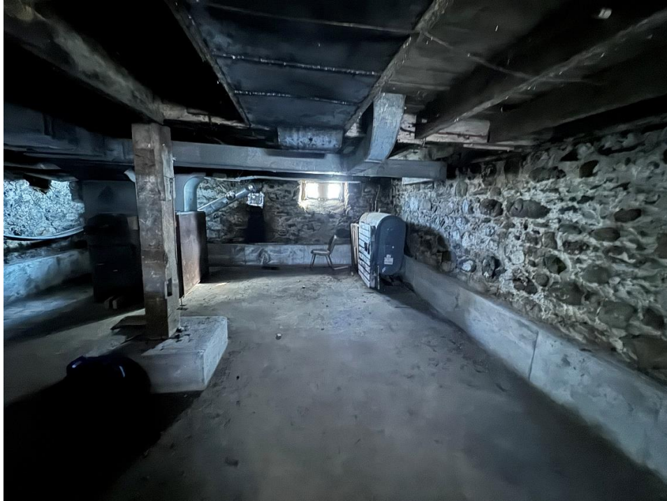
Photo #13: Basement, underpinning, rubble foundation wall
