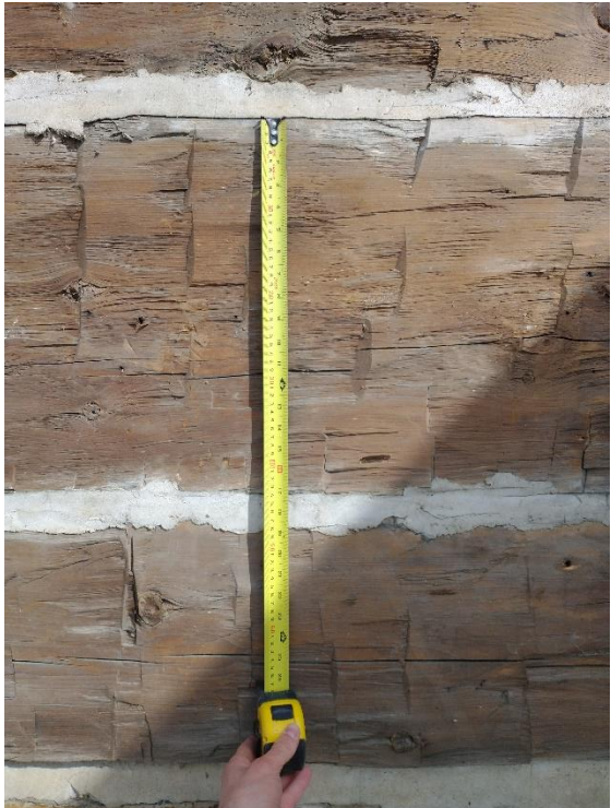
Photo #10: Wall log depth measurement
