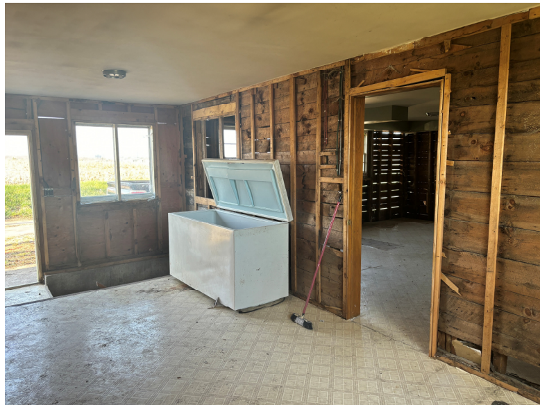
UTILITY ROOM 2- STOREY WALL
