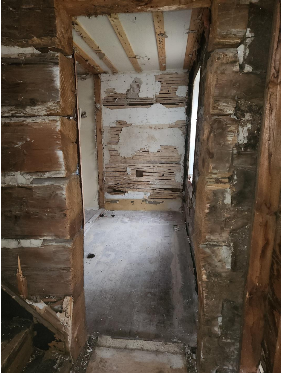
Photo #19: Northwest corner washroom door opening.
