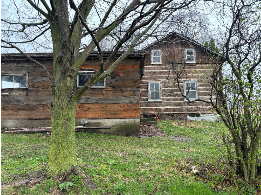
Photo #4: West Elevation (exterior finishes removed)
