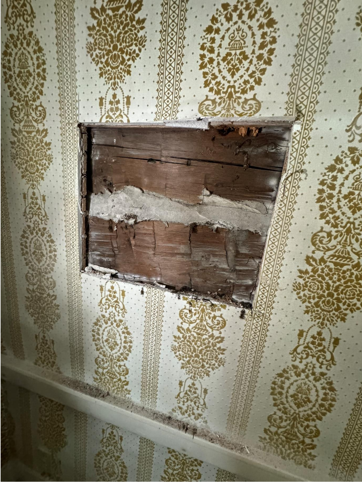
Photo #12: Exposed portion of wall from interior
