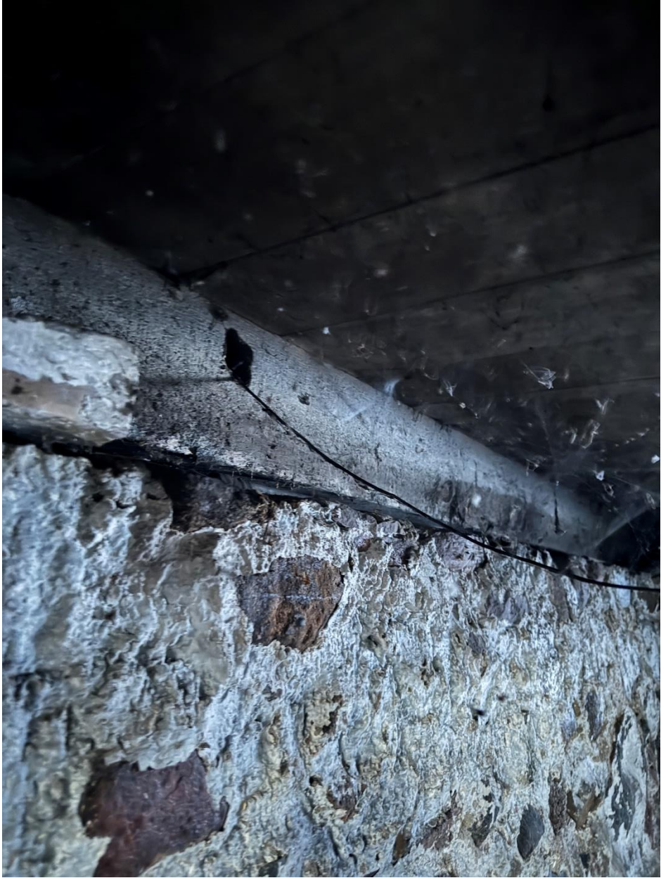
Photo #16: End bearing condition over rubble wall.
