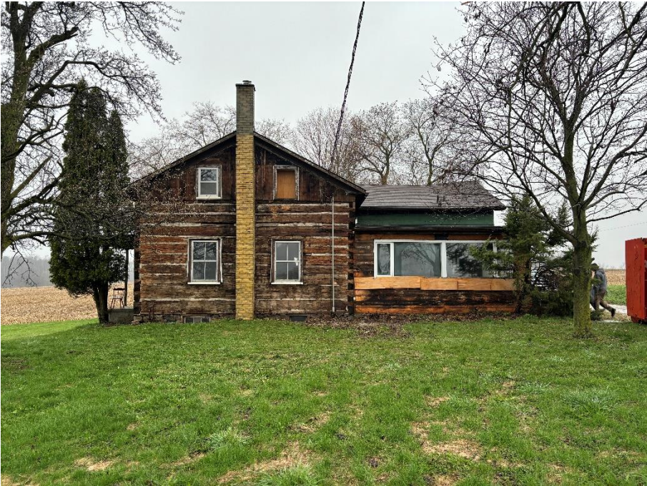
Photo #2: East elevation (exterior finishes removed)
