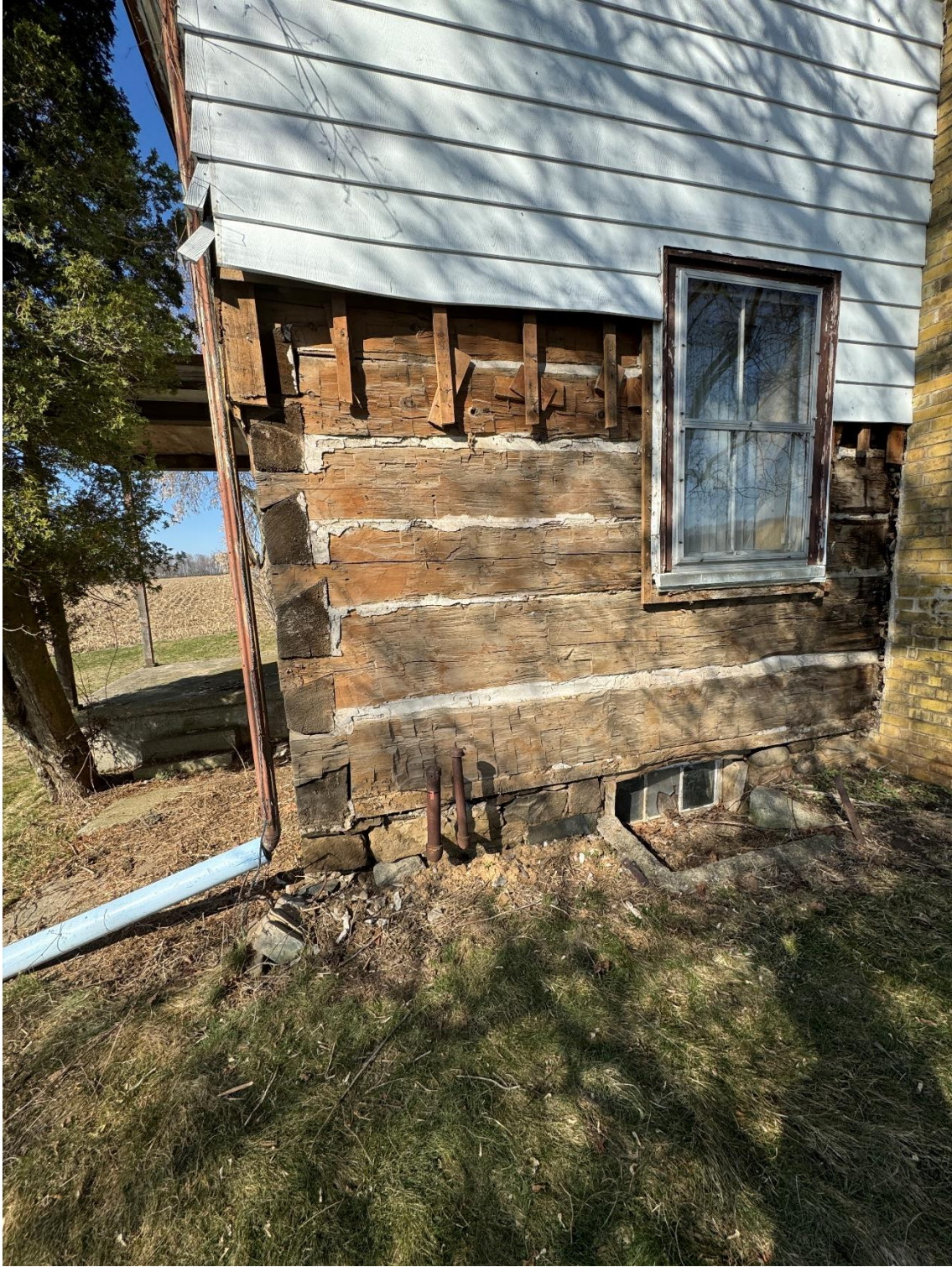
Photo #5: Exterior log wall and dutchman / finger joint corner from east elevation
