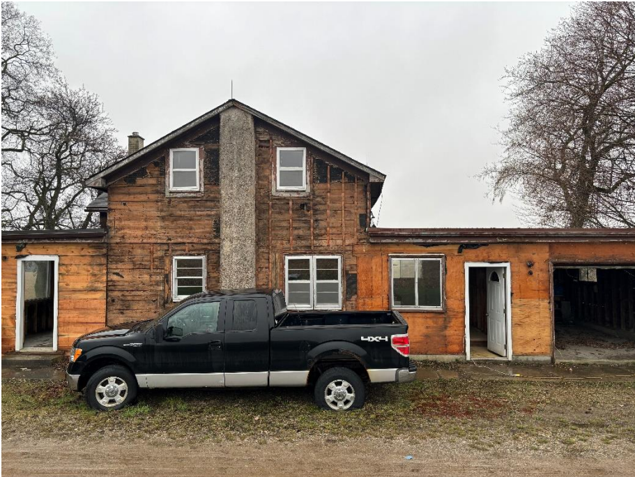
Photo #1: North elevation (exterior finishes removed)
