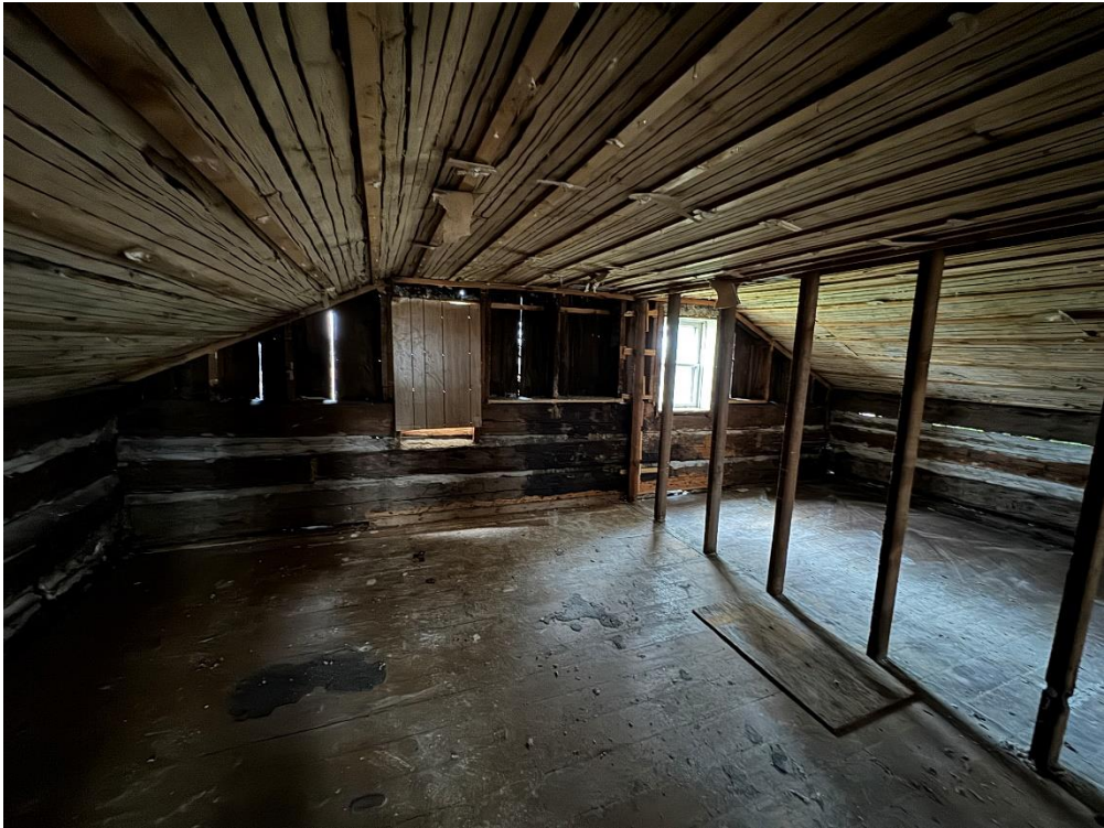
Photo #18: Roof framing finishes removed.
