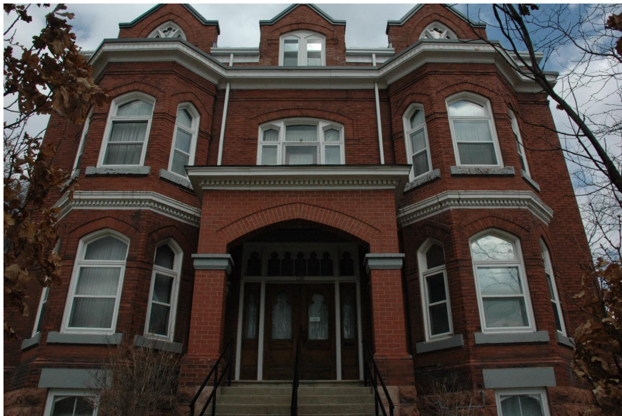
Figure 2. Façade fronting onto 56 Duke Street West.
