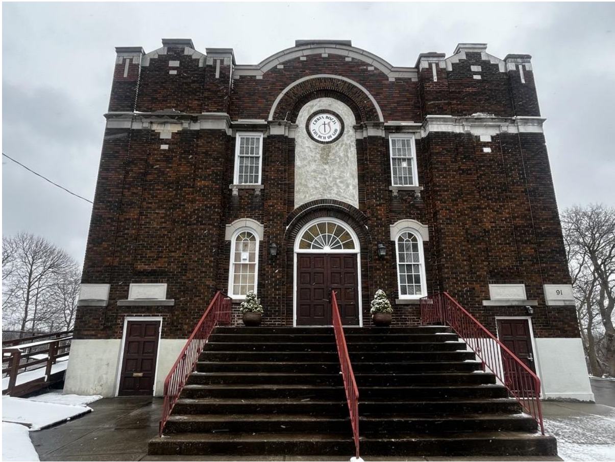
Figure 2: Front Façade of Subject Property (2024)
