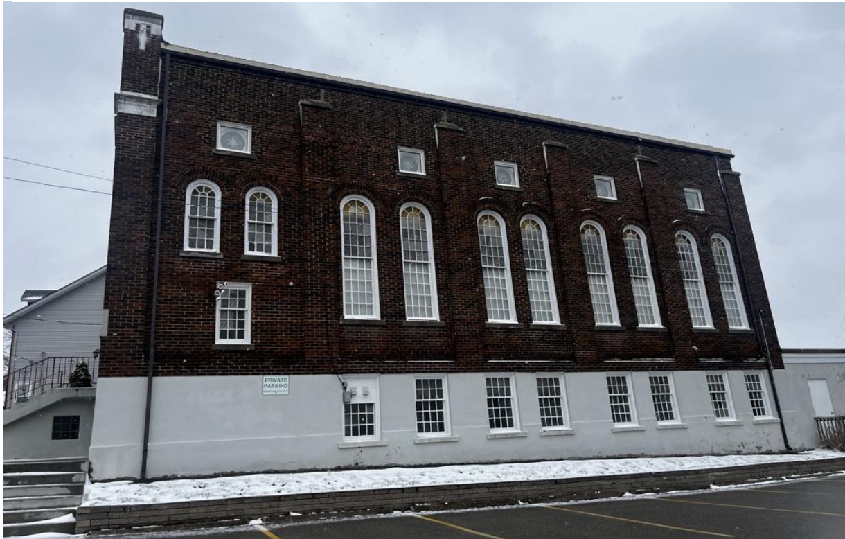
Figure 3: North Side Façade of Subject Property (2024)
