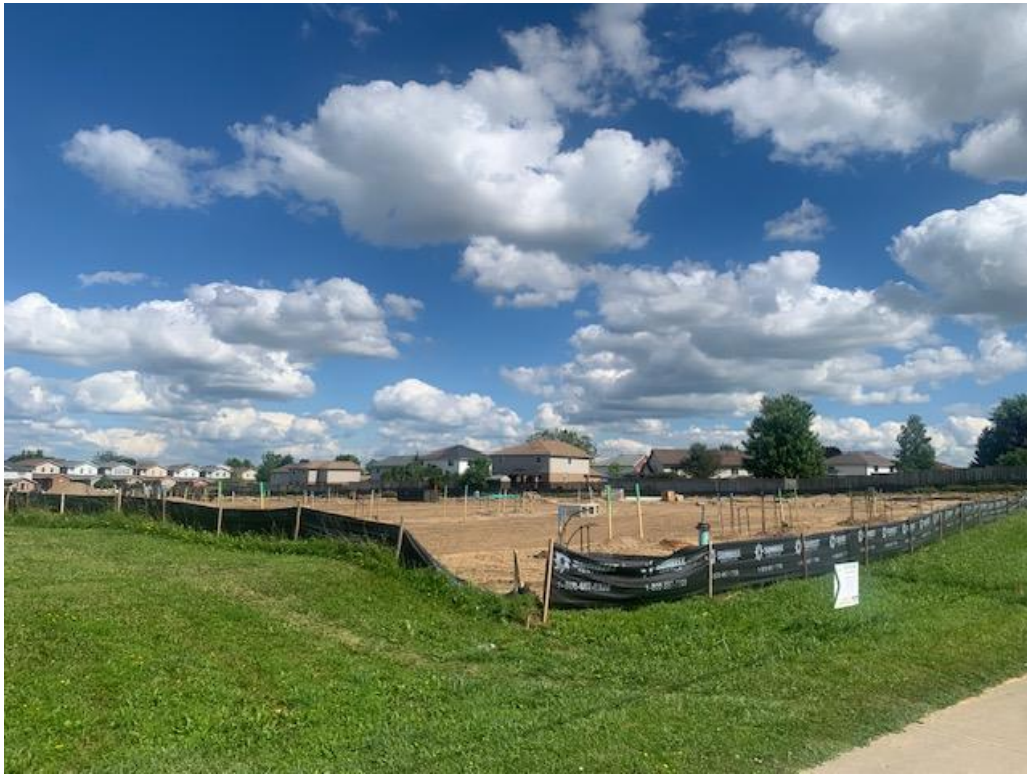
Figure 3: Existing Site Conditions at 1188 Fischer Hallman Road
