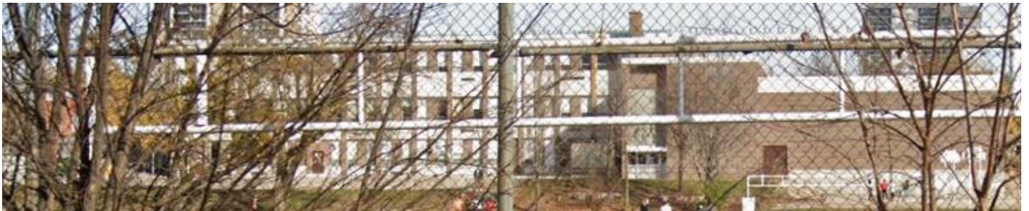
Rear Elevation (South Façade) – 107 Courtland Avenue East
