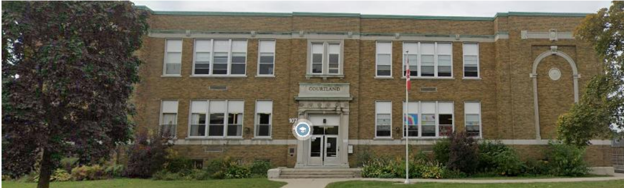
Front Elevation (North Façade) – 107 Courtland Avenue East
