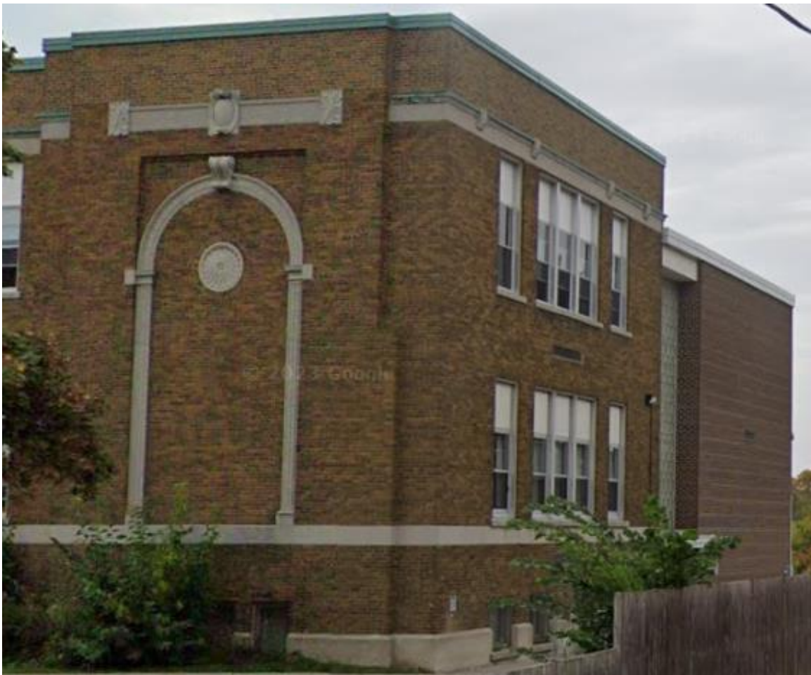
Side Elevation (West Façade) – 107 Courtland Avenue East
