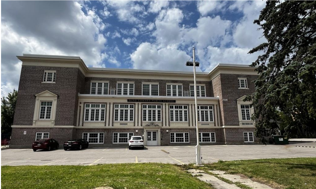
Figure 2: Front Facade of Subject Property
