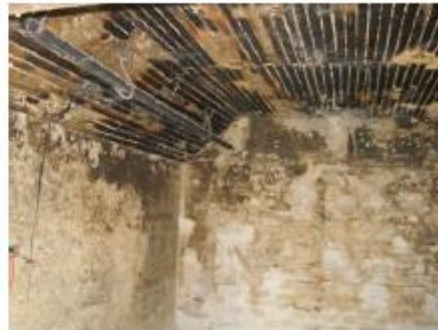
Figure 70: Interior view of smoke house
