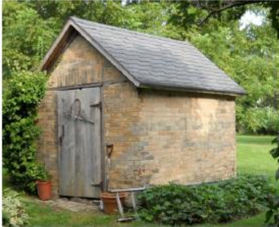
Figure 69: Smoke house, 1478 Trussler Road
