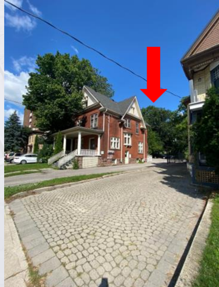
Location of proposed addition highlighted by red arrow.
