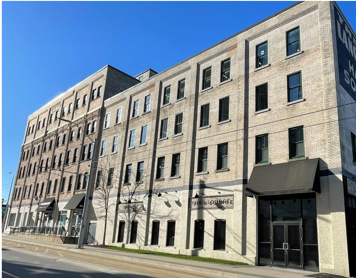
Figure 3: Front Elevation (North Façade) – Former Administration and Tan Yard Buildings of the Lang Tanning Co.
