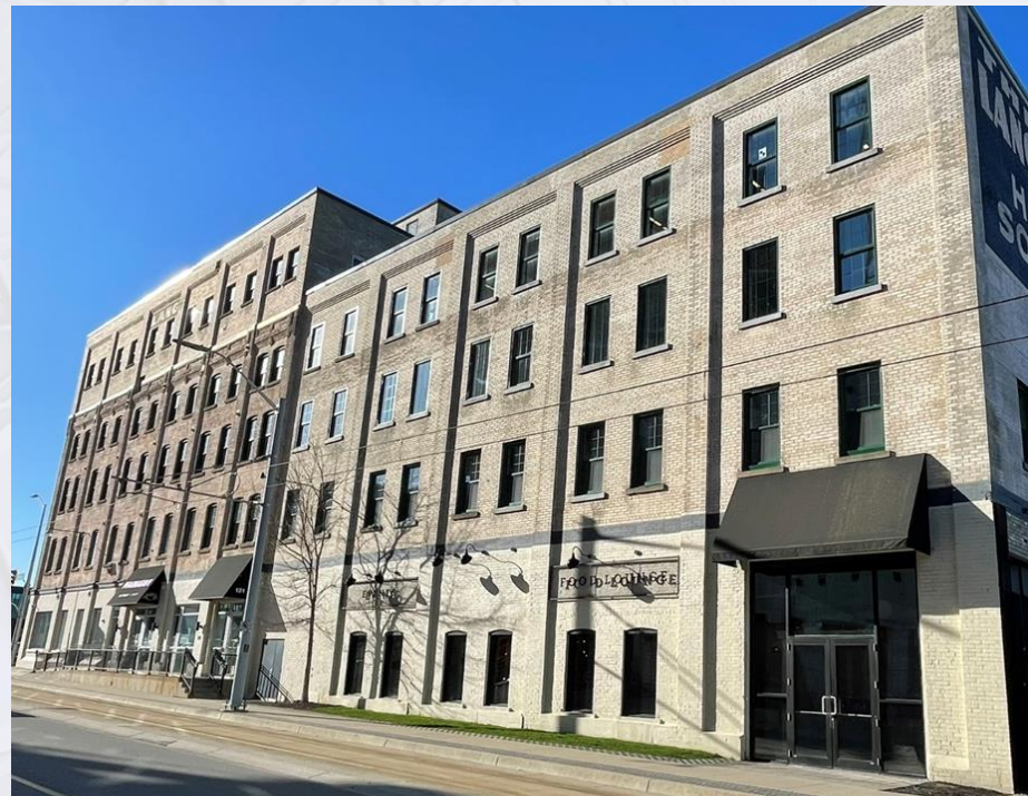
Former Administration and Tan Yard Buildings of the Lang Tanning Co.
