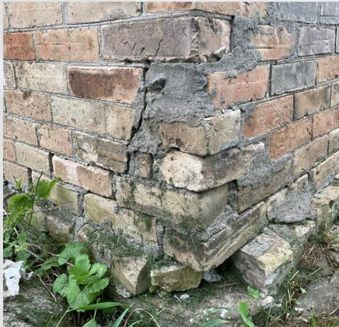
Photograph showing missing bricks, step cracks and inappropriate mortar repairs
