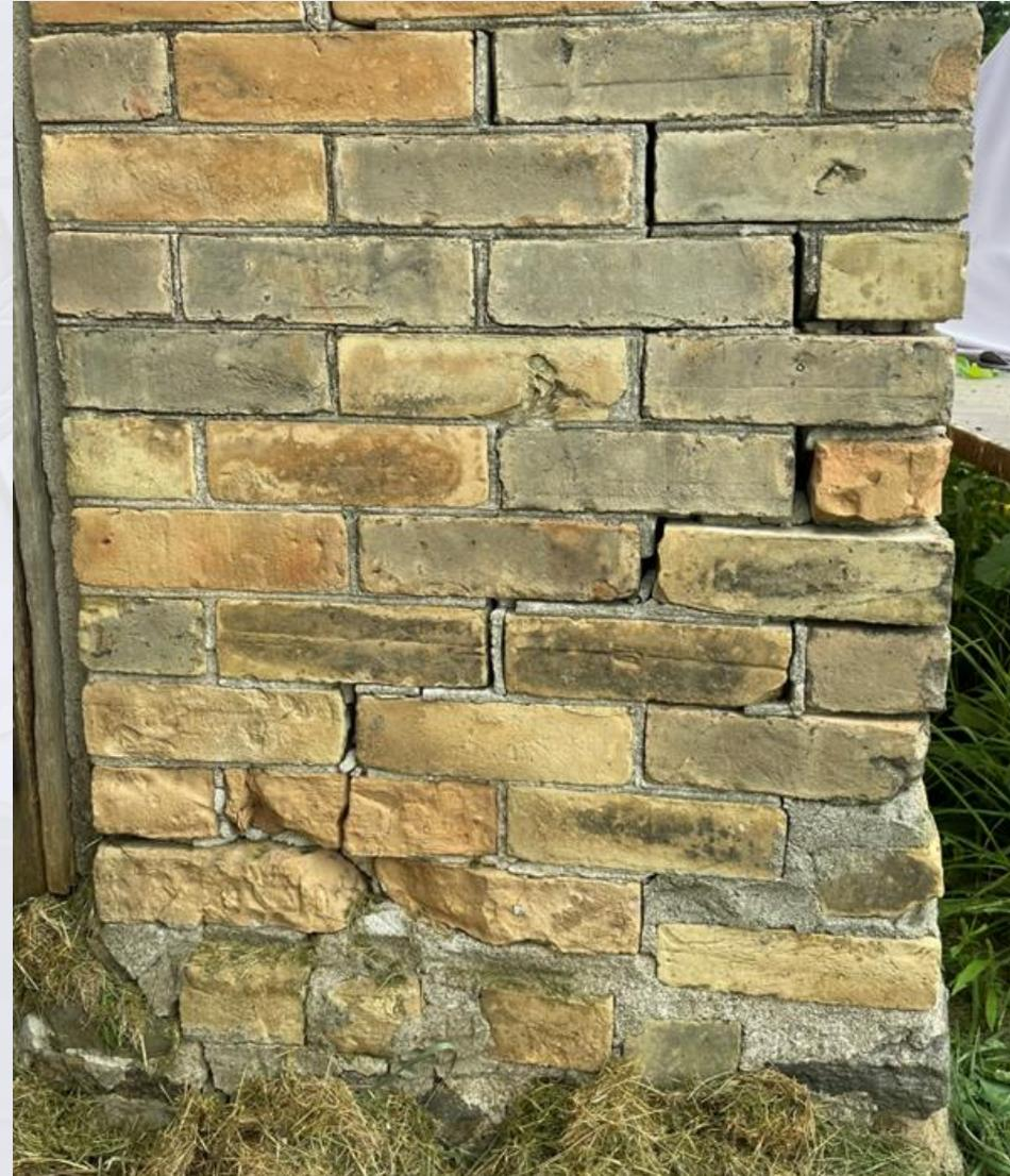
**Photograph showing step crack and spalling bricks**
