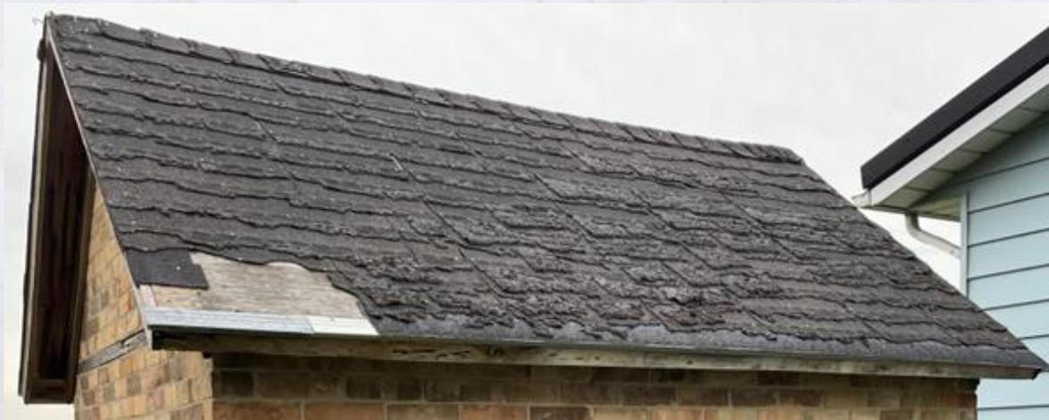
Photograph showing deteriorated/missing asphalt shingles
