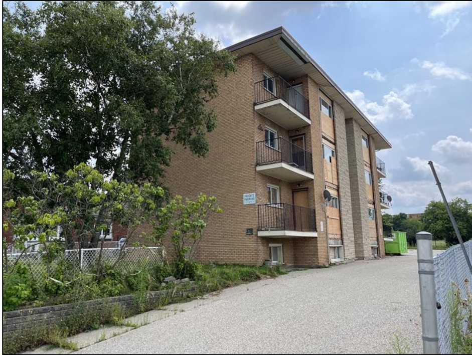
Figure 2: View of Existing Vacant Multiple Dwelling Building (August 1, 2024)
