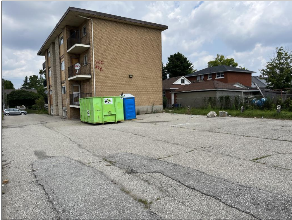
Figure 4: View of Existing Rear Parking Area (August 1, 2024)
