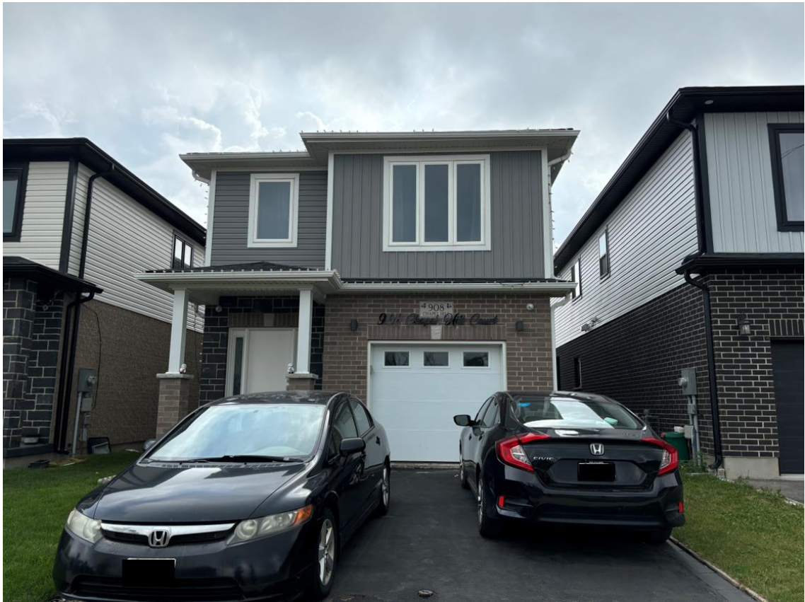
Figure 5 – Site Photo of 908 Chapel Hill Court.
