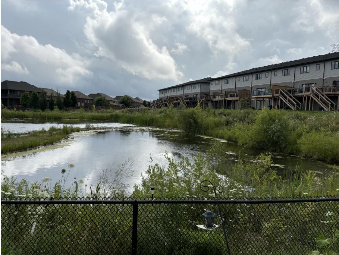
Figure 7 – Existing Stormwater Management Pond abutting the rear of the property.
