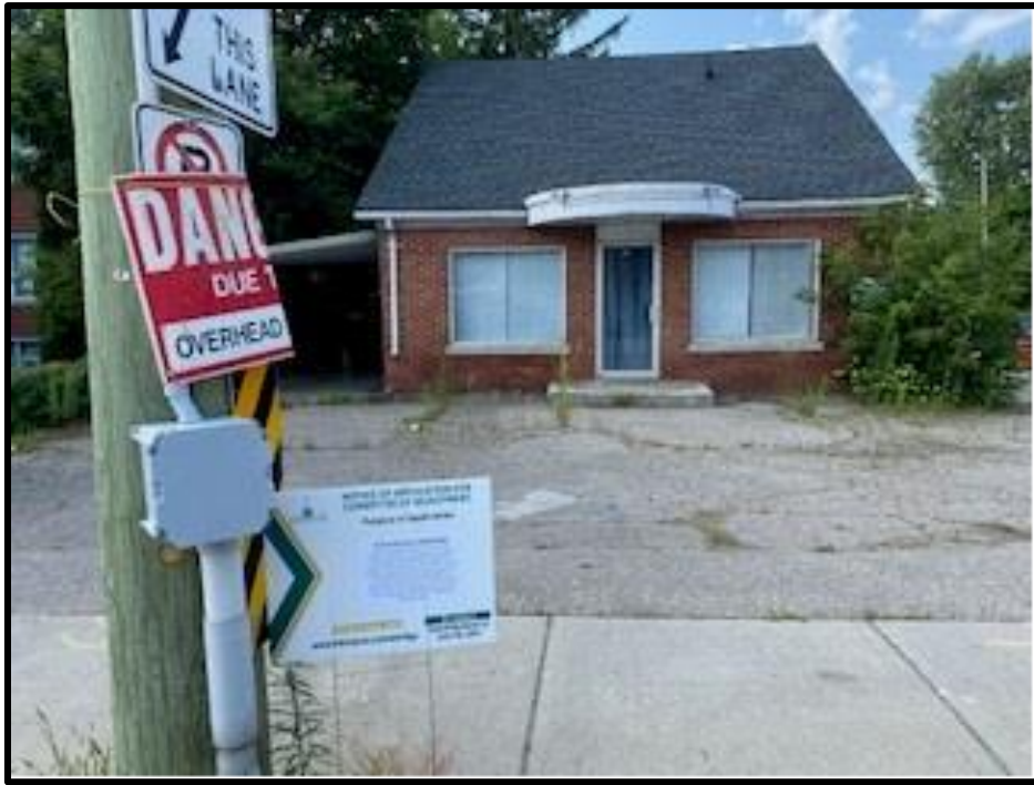
Figure 2 - Photo of 570 Frederick Street
