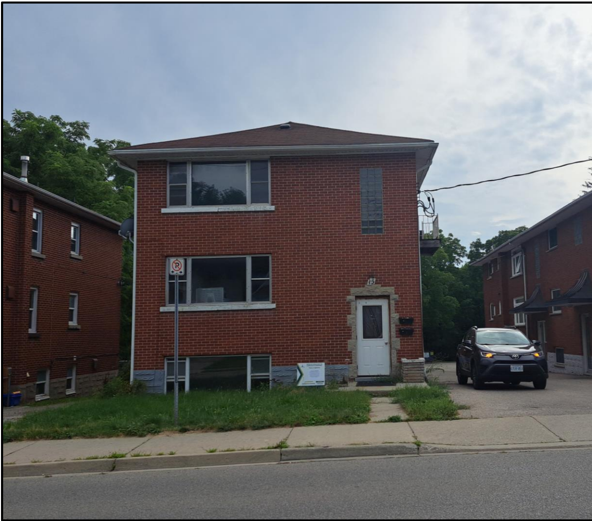
Figure 4: The front view of the subject property from Strange Street
