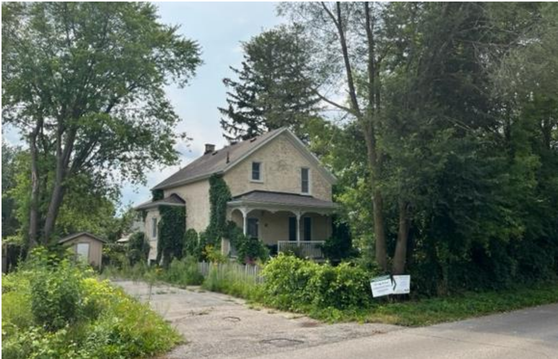
Figure 3: Existing single detached dwelling at 62 Gage Avenue to be demolished
