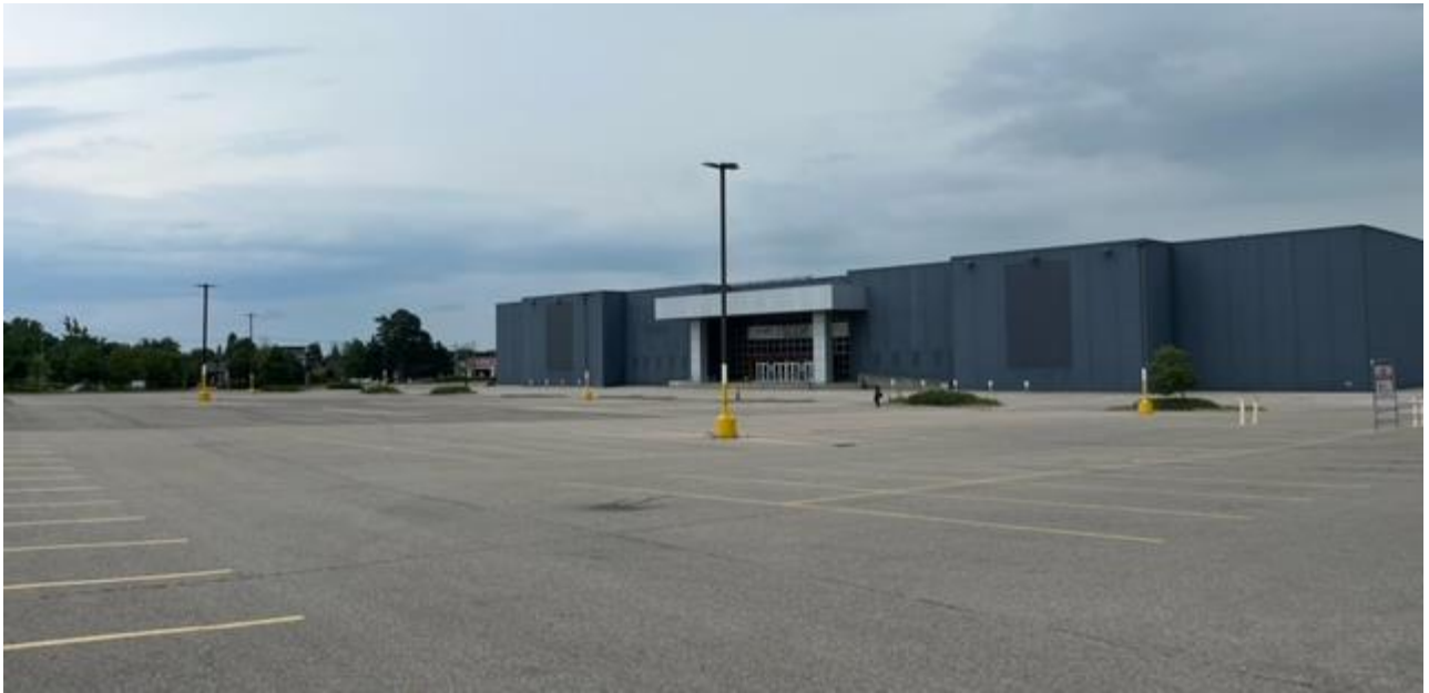
Figure 5: Existing building and existing conditions
