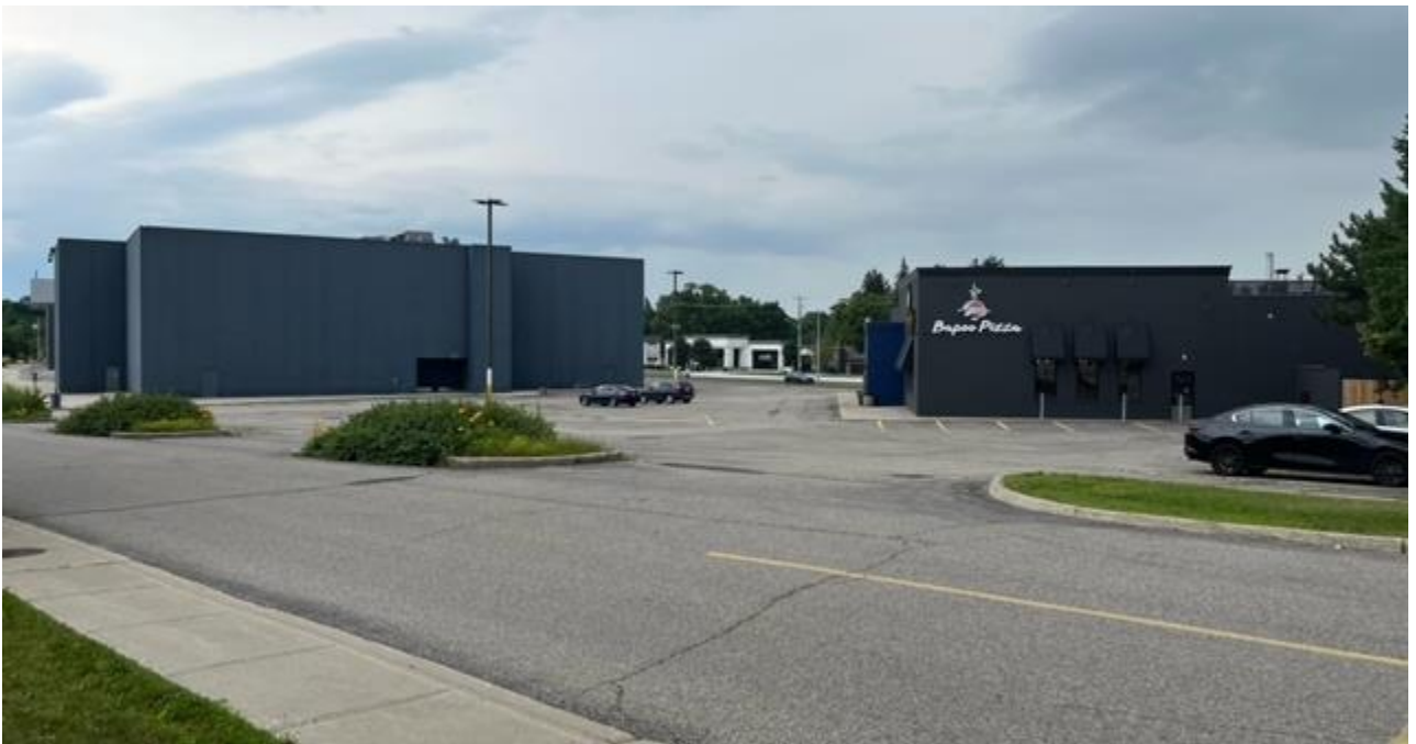
Figure 6: Existing buildings and existing conditions
