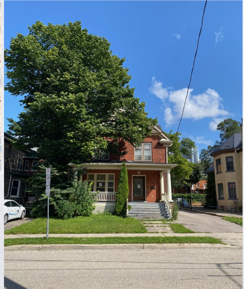
Front Façade of 99 College Street
