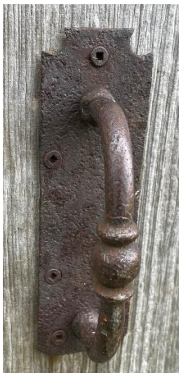
Detail of Door Hardware on Front Elevation (South Façade) – 1478 Trussler Road
