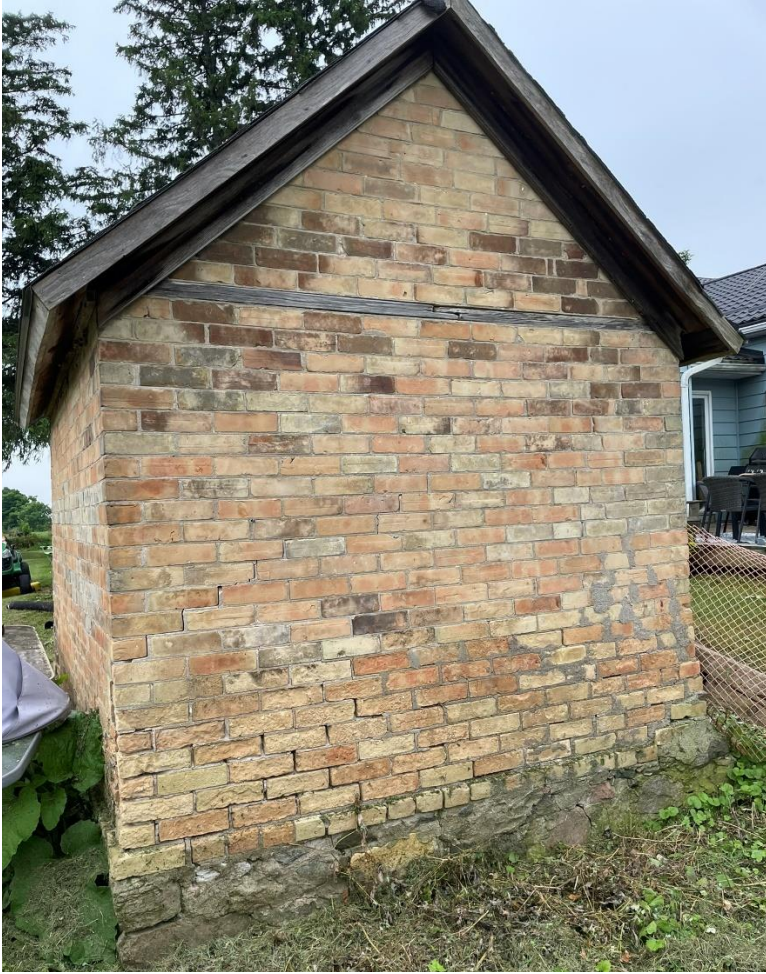
Rear Elevation (North Façade) – Smoke House at 1478 Trussler Road
