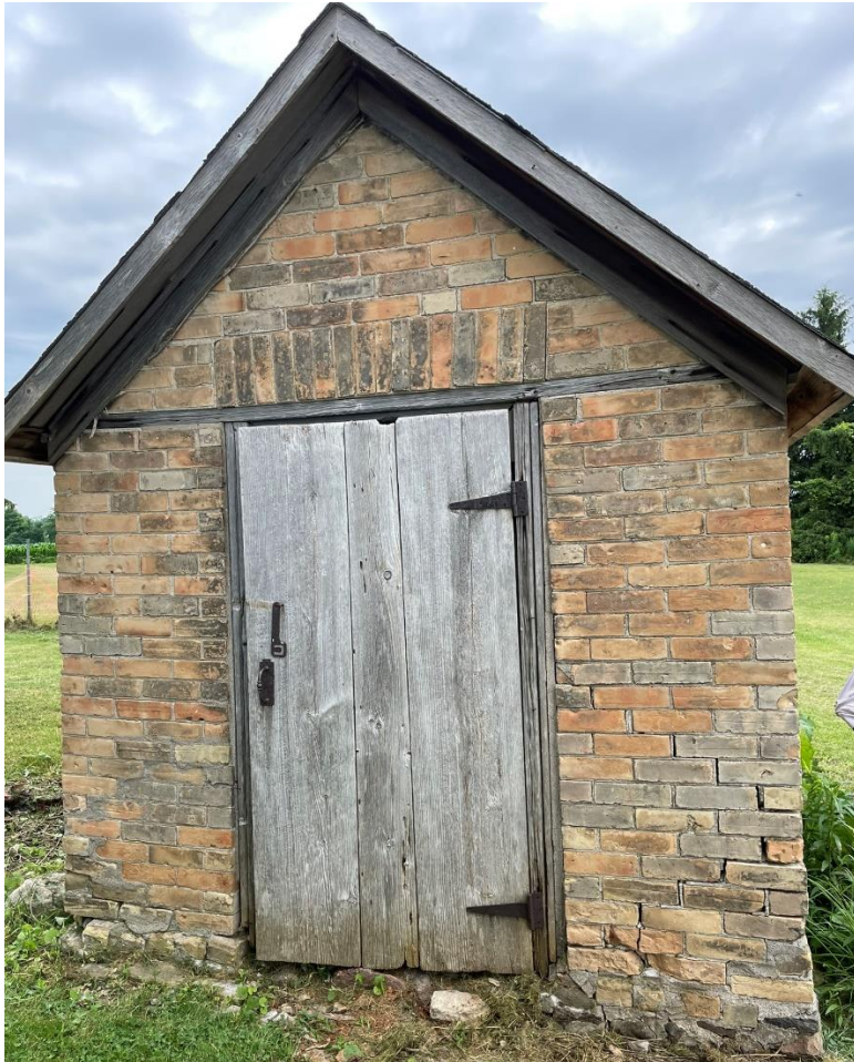
Front Elevation (South Façade) – Smoke House at 1478 Trussler Road
