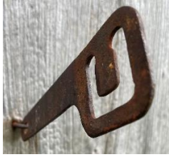
Detail of Door Hardware on Front Elevation (South Façade) – 1478 Trussler Road
