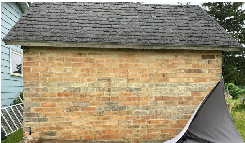
Side Elevation (East Façade) – Smoke House at 1478 Trussler Road
