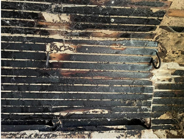
Interior Photograph of Charred Wood Slats and Metal Hooks inside the Smoke House – 1478 Trussler Road
