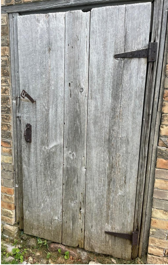
Detail of Door on Front Elevation (South Façade) – 1478 Trussler Road
