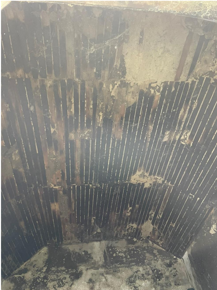
Interior Photograph of Charred Wood Slats inside the Smoke House – 1478 Trussler Road
