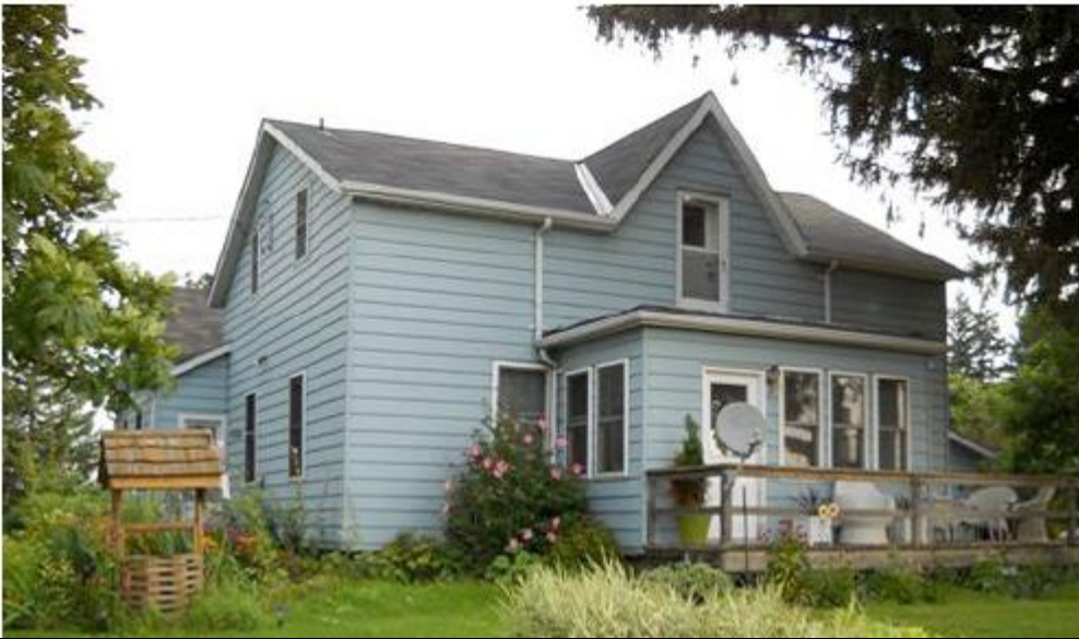
Front Elevation (South Façade) – 1478 Trussler Road
