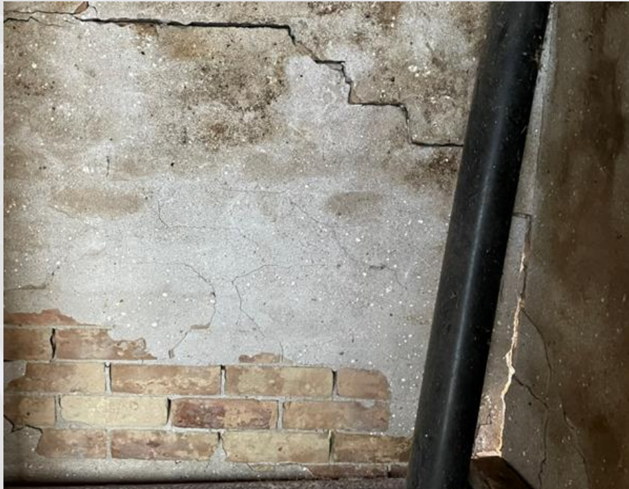
Photograph showing major cracks through the parging and mortar where you can see through the smoke house
