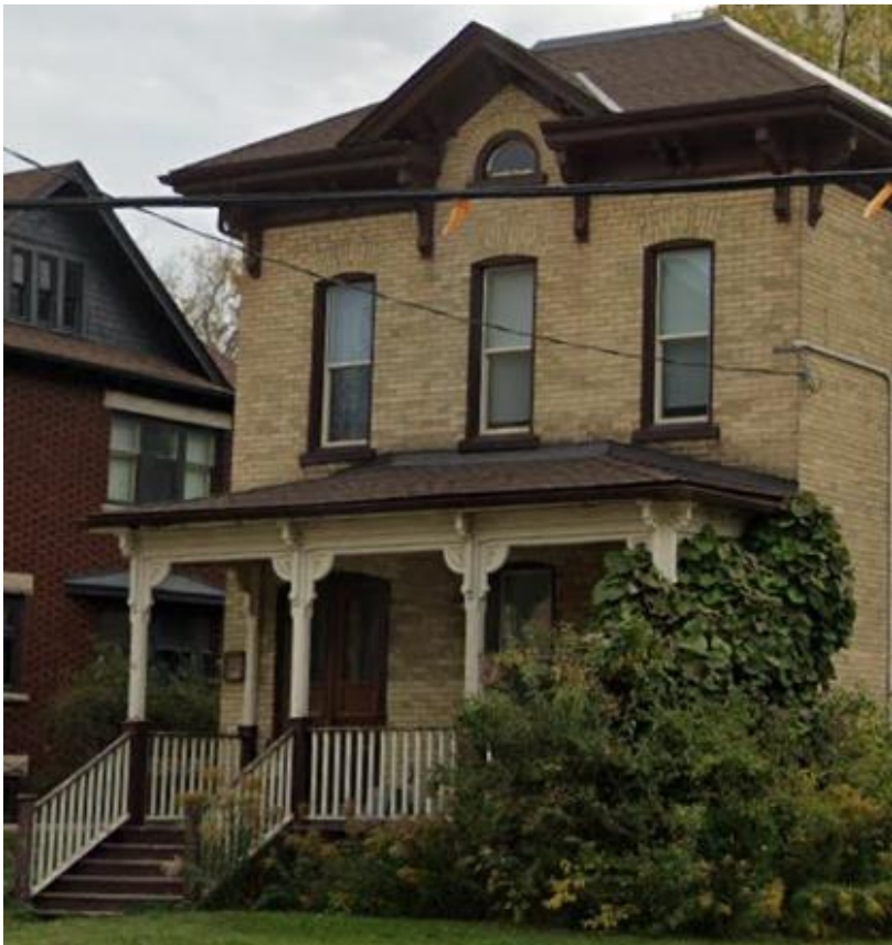
Front Elevation (North Façade) – 83 Benton Street
