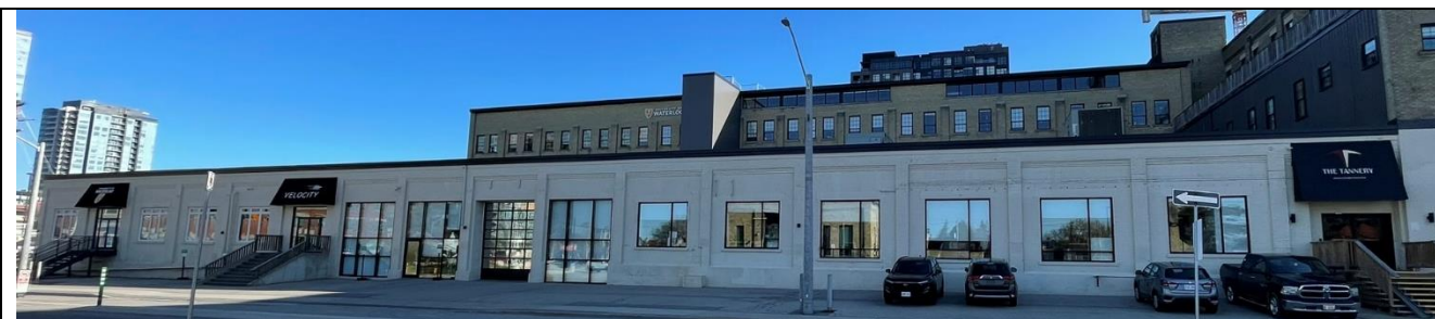
Rear Elevation (South Façade)
