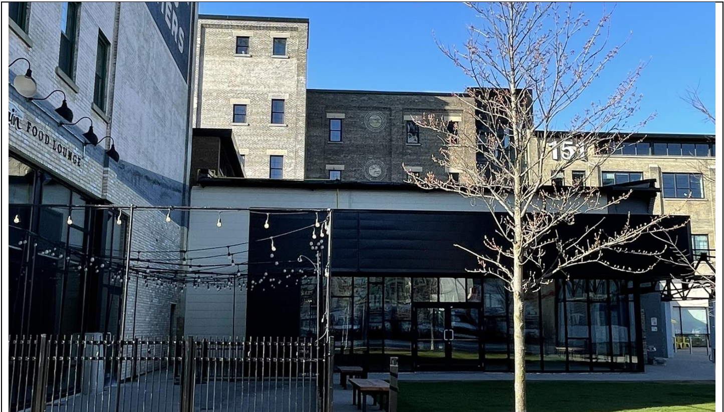
Front Elevation (North Façade) – New Additions and the Former Leech House of the Lang Tanning Co.
