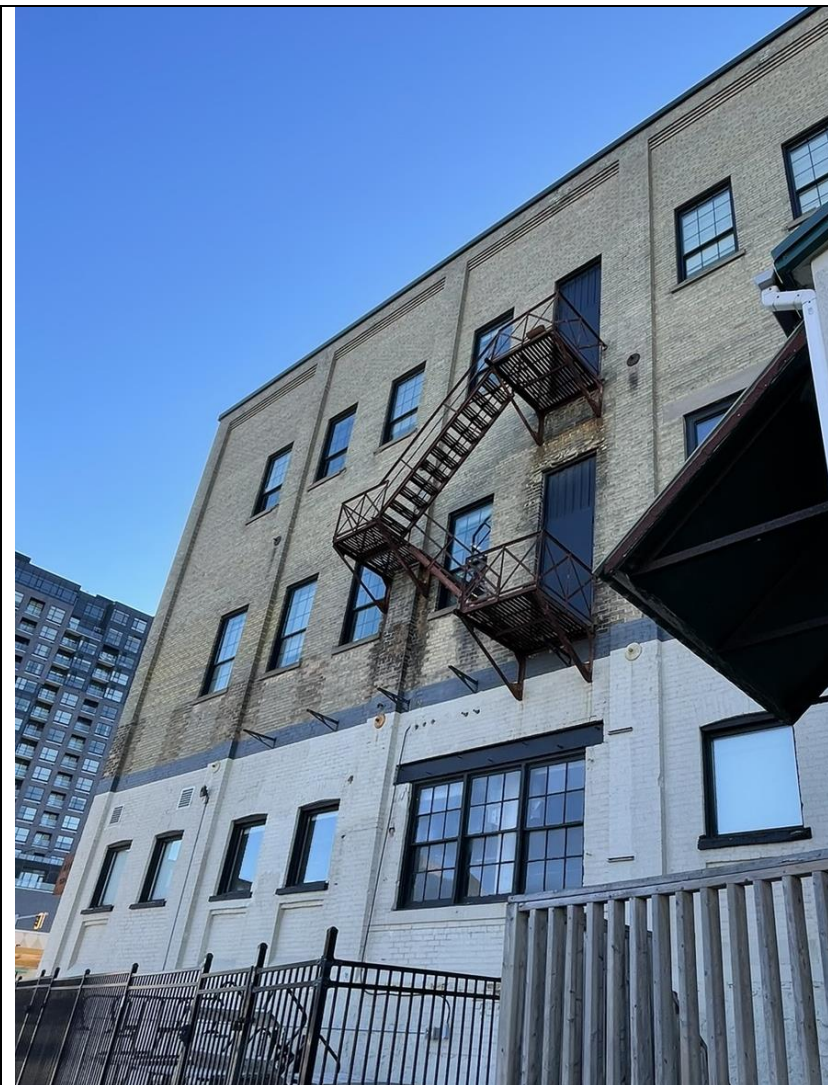
Side Elevation (West Façade) – Former Beam and Storage House of the Lang Tanning Co.
