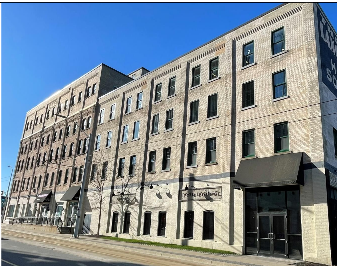
Front Elevation (North Façade) – Former Administration and Tan Yard Buildings of the Lang Tanning Co.
