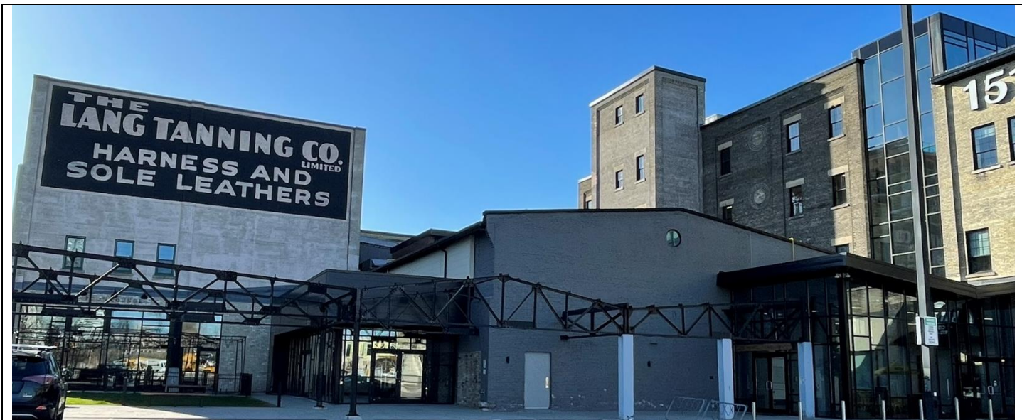
Side Elevation (West Façade) – Former Tan Yard Building (left) and New Additions (right) of the Lang Tanning Co.
