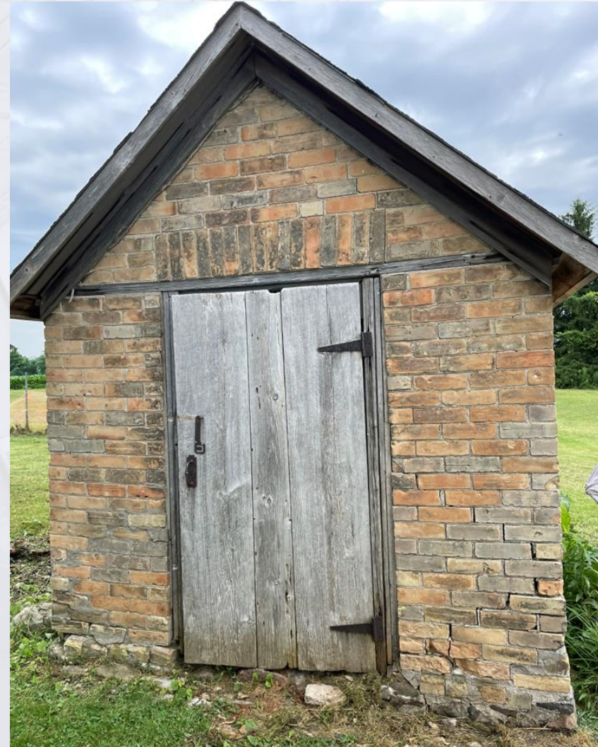
Front Elevation: Smoke House
