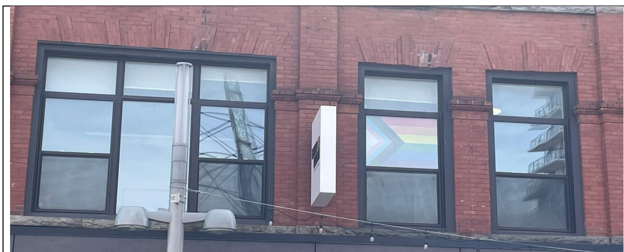
Detailing of second-storey with a ribbon of three windows in the first bay; two flat head window openings in the second bay; rectangular transoms; and, 1/1 hung window design with brick voussoirs and continuous stone sills
