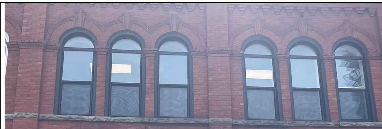
Detailing of third-storey semi-circular window openings; semi-circular transom design; 1/1 hung window design featuring decorative brick hood moulds with keystones and continuous stone sills
