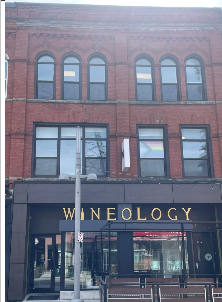
Front Elevation (North Façade) – 87-91 King Street West
