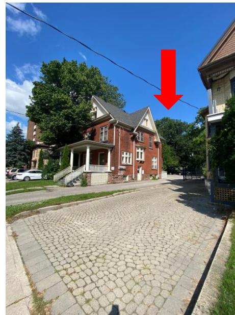
Figure 9. View from the street. Approximate location of the addition highlighted by red arrow and will be highly visible from the street.
