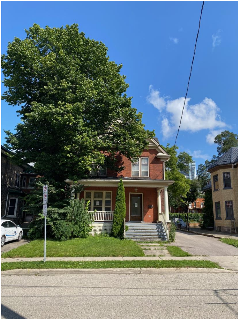
Figure 2. Front Elevation of subject property
