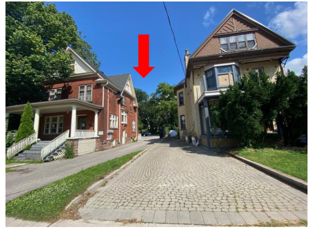
Figure 11. View from the street. Approximate location of the addition highlighted by red arrow and will be highly visible from the street.
