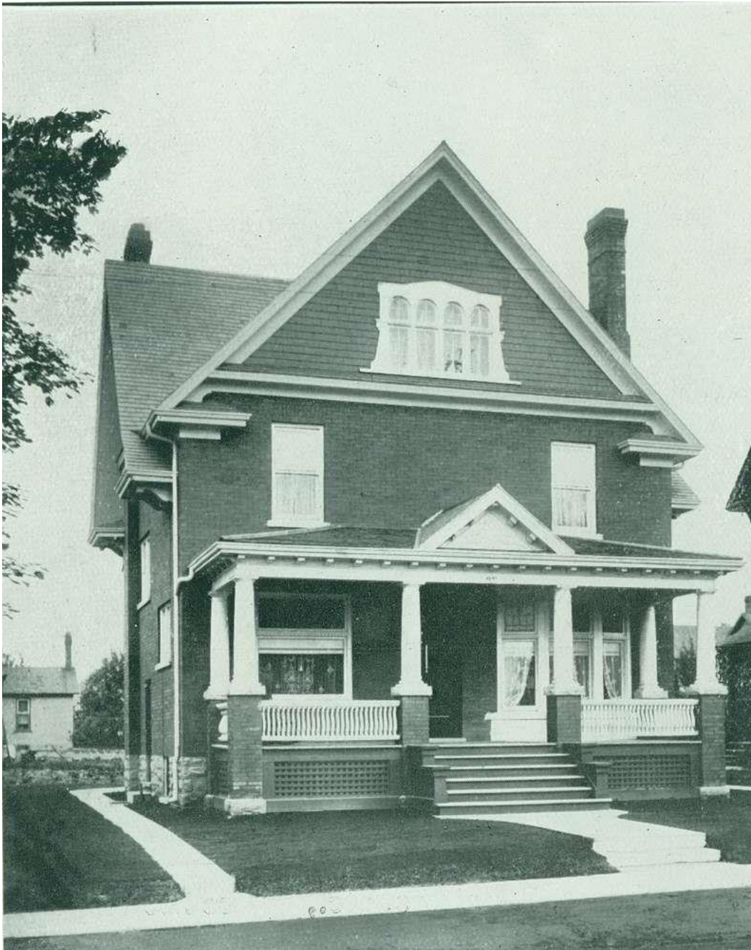
Front Elevation (North Façade) – Historic Photograph circa 1912
