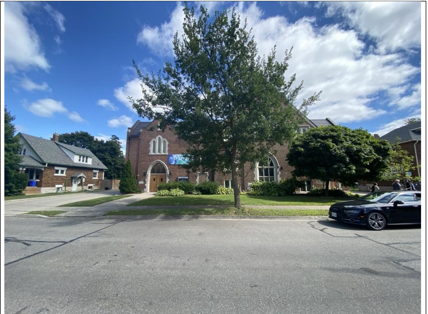
Stirling Avenue Mennonite Church – Front Facade
