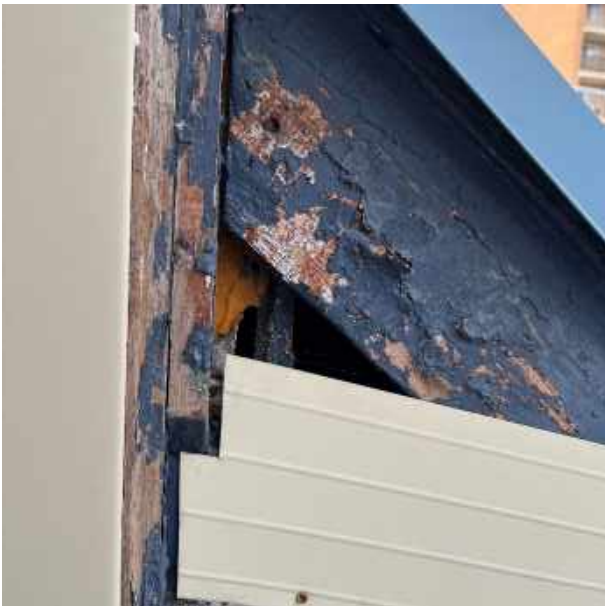
73 Benton St (Upper Unit) Exposed Eaves
