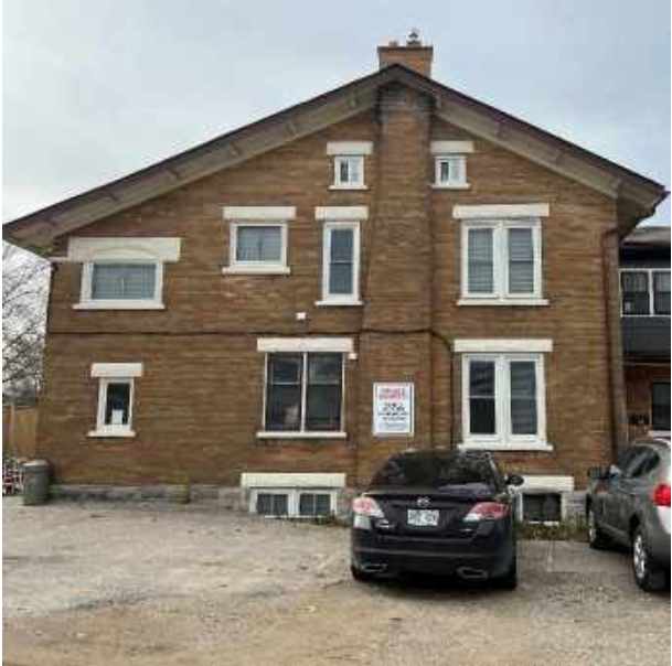
69 Benton St North (Side) Facade
