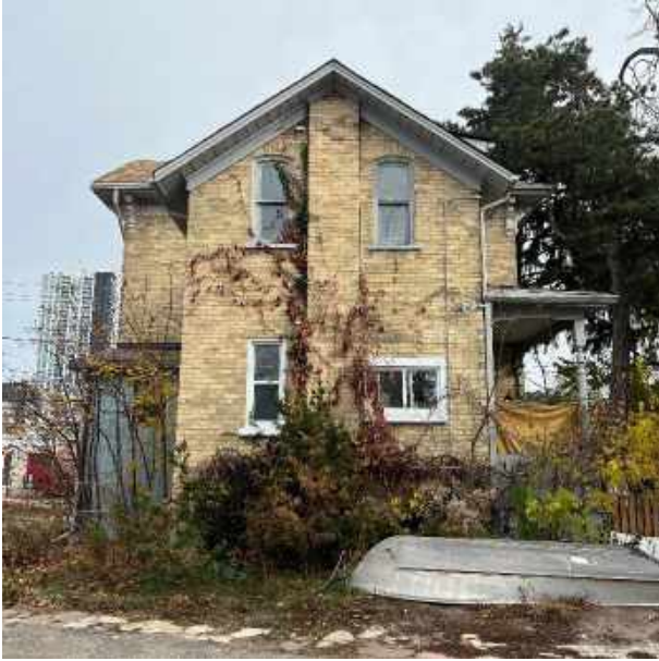
51 Church St South (Rear) Facade
