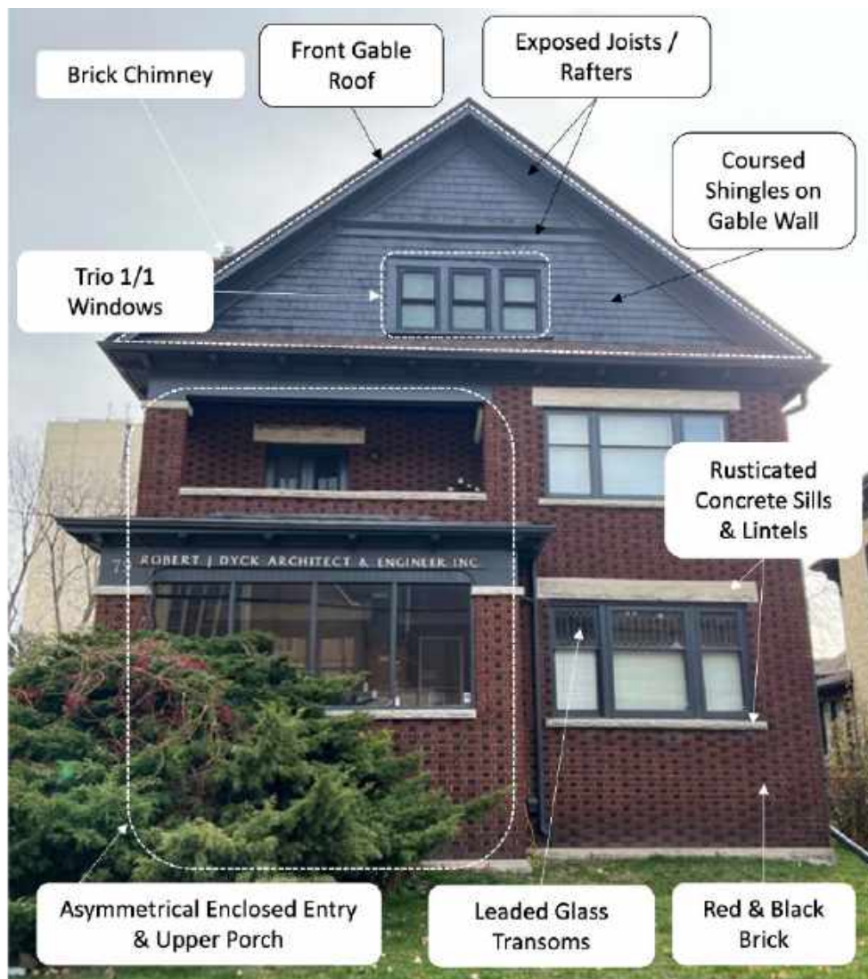
Figure 79 - Visual of Exterior Attributes, 79 Benton Street
