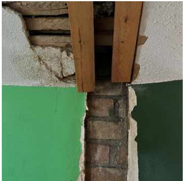
Benton St (Upper Unit) Exposed Brick & Lath & Plaster
