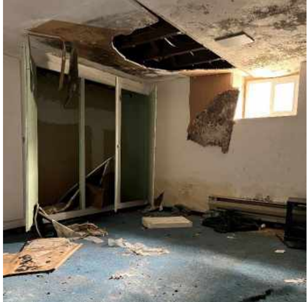
73 Benton St (Basement) Mould
