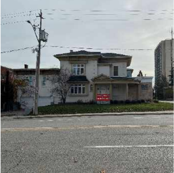
51 Benton St Italianate Structure
