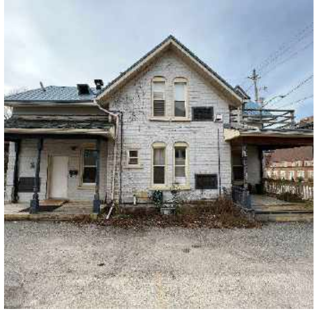
73 Benton St North (Side) Facade
