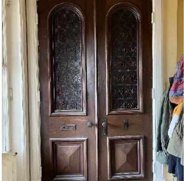
51 Church St (Upper Unit) Original Front Entrance Door
