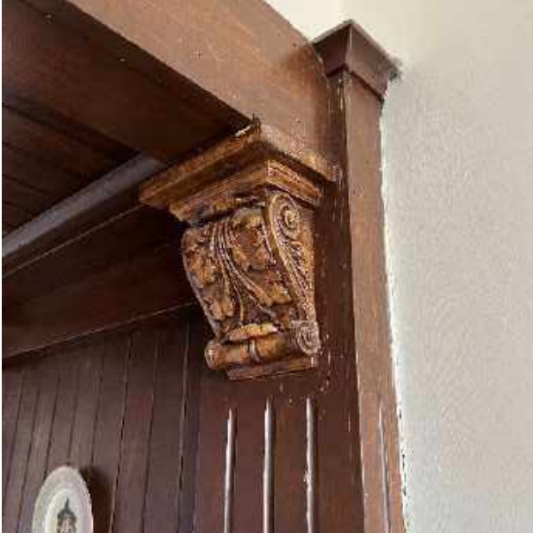
51 Church St (Upper Unit) Decorative Woodwork
