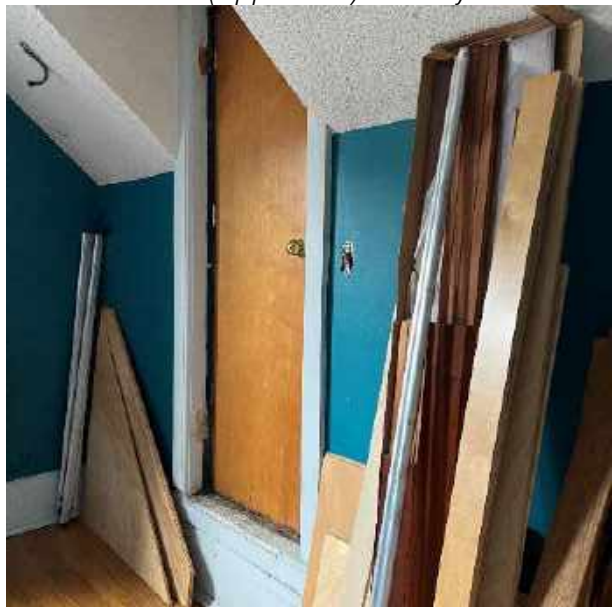
73 Benton St (Upper Unit) Balcony Access
