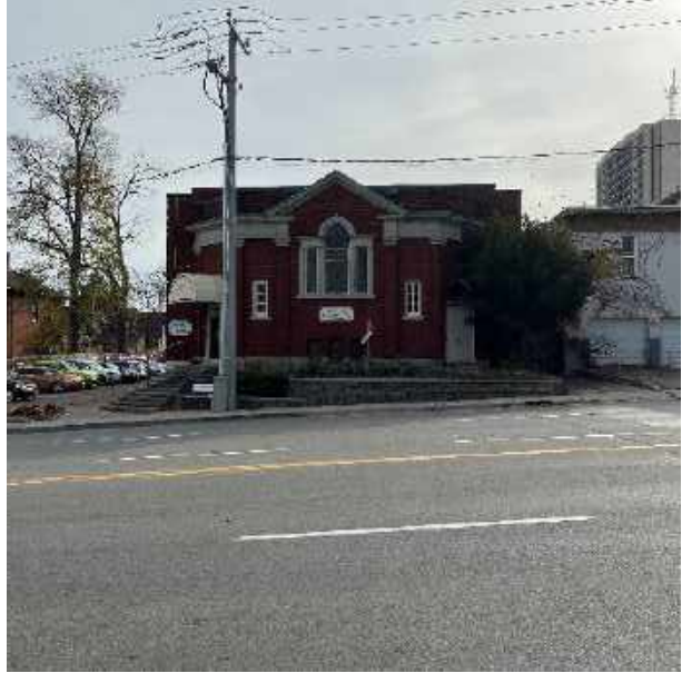
43 Benton St (MacKenzie King Manor) North of Subject Lands
