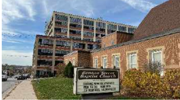
Benton St Baptist Church & Arrow Lofts Interface
