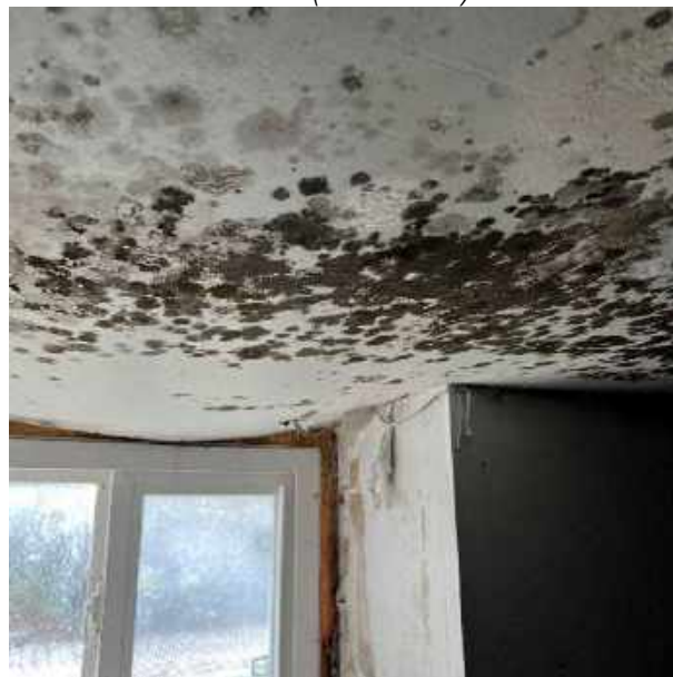
73 Benton St (Basement) Mould
