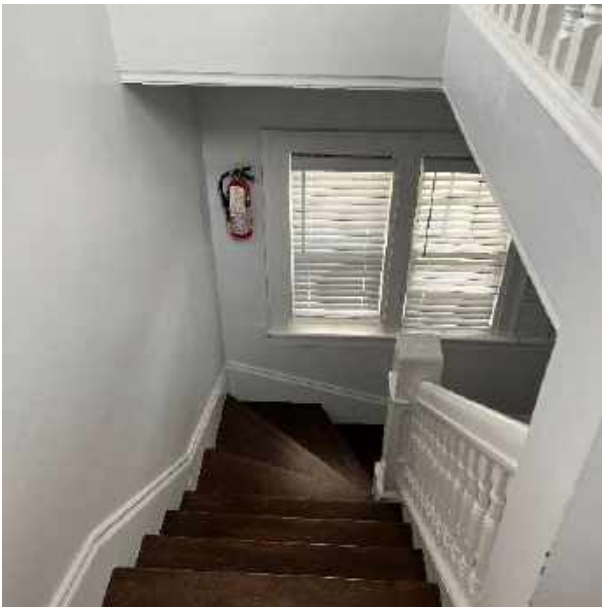
69 Benton St Staircase between Upper Unit and Ground Floor
