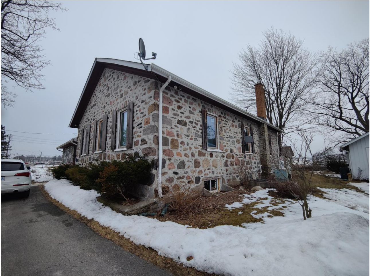
Figure 2. North and West elevation of the original Williamsburg Schoolhouse.
