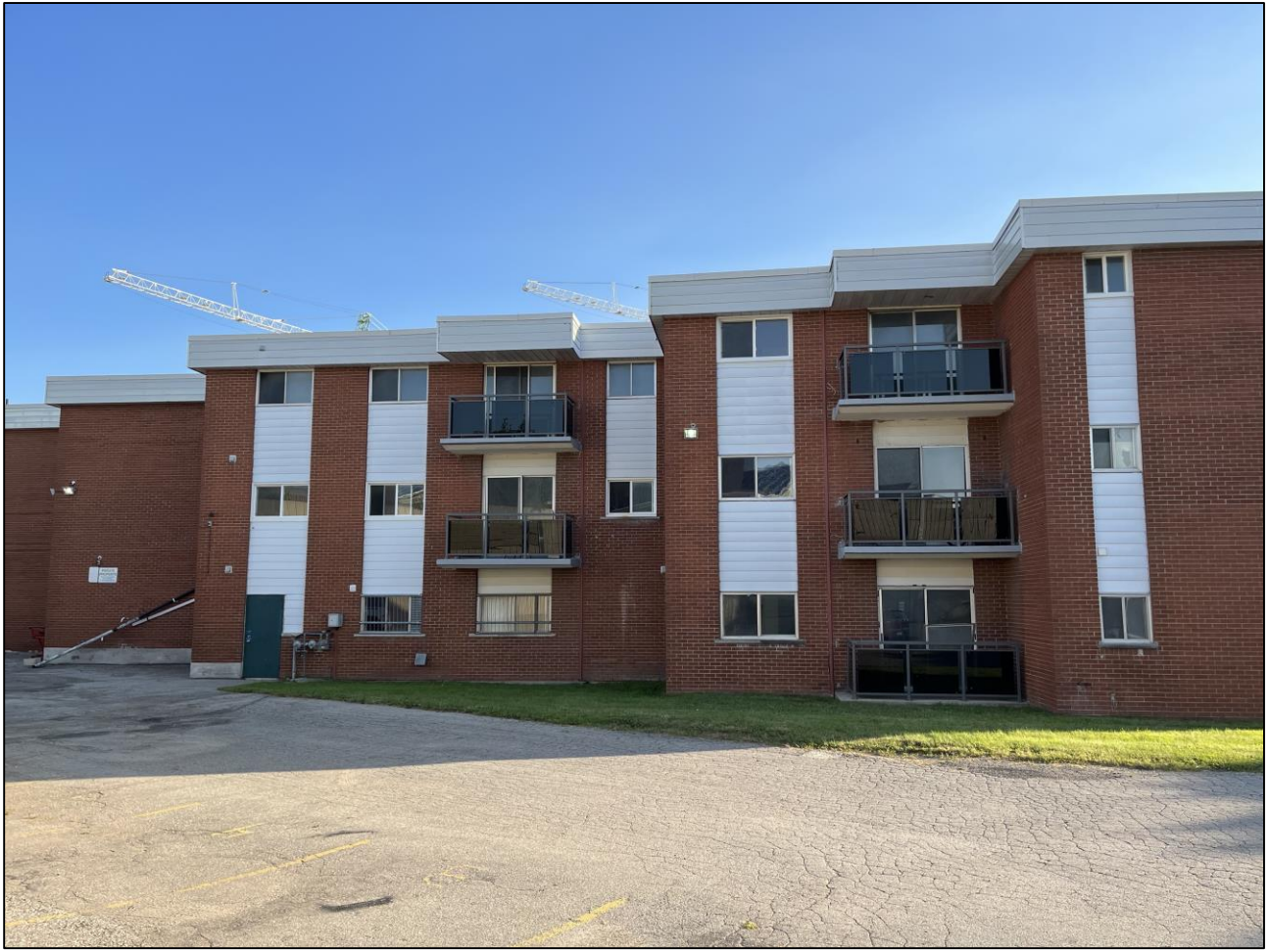
Figure 4: View of Rear of Existing Building (September 3, 2024)
