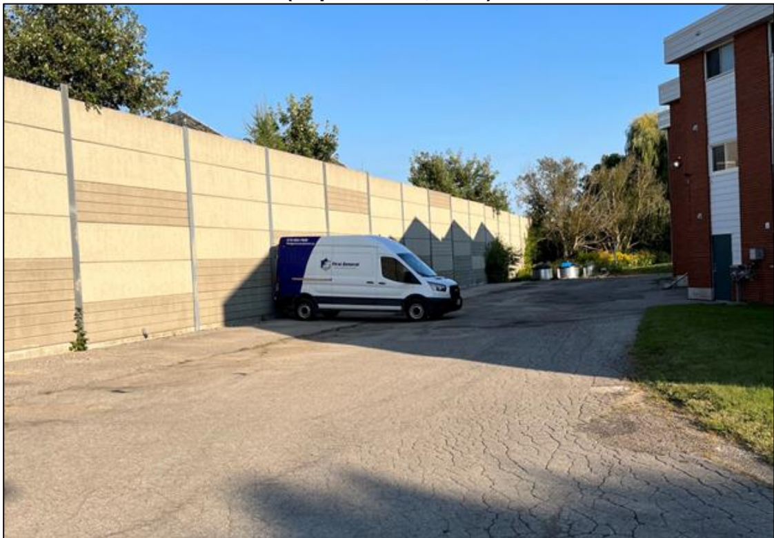
Figure 3: View of Existing Parking Area and Noise Wall (September 3, 2024)
