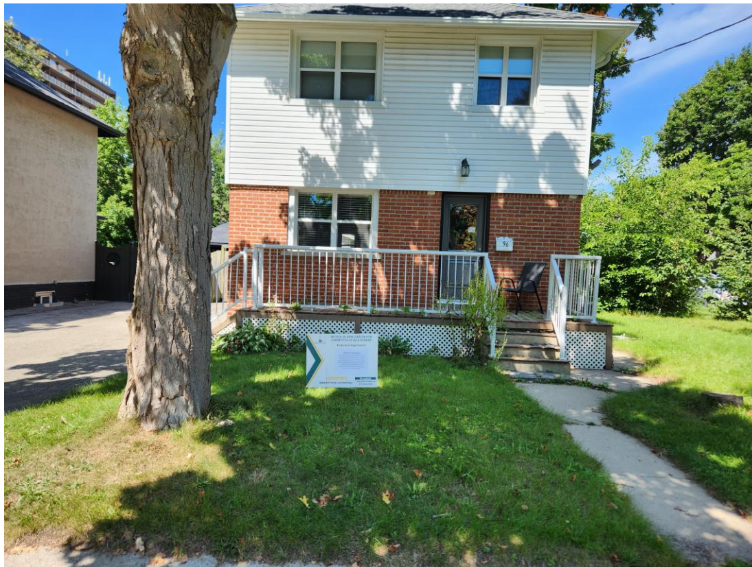
Figure 4: Front of Existing House (Wood Street Façade)
