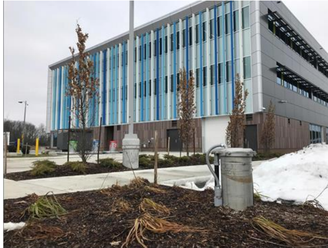
Figure 12: Open Loop Well Installation in Waterloo 6
