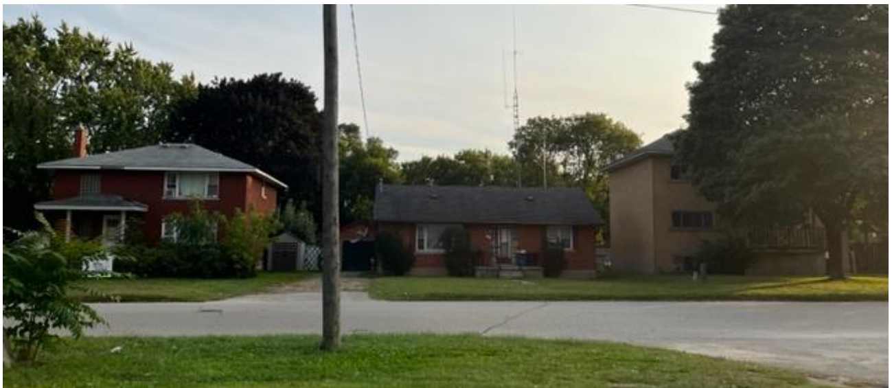
Figure 2 – Existing buildings at 9-27 Turner Avenue
