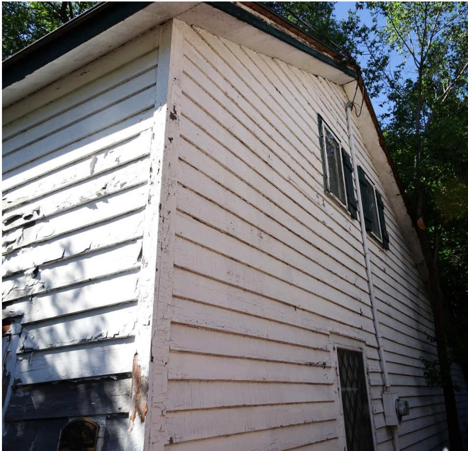
Photo 4. Side (West) Elevation in 2020
