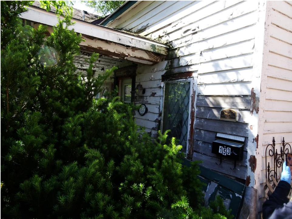
Photo 1. Front (North) Elevation in 2020
