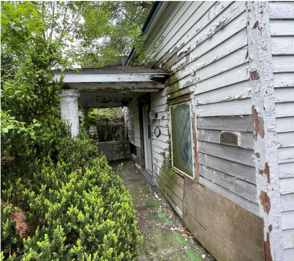
Photo 5. Front (North) Elevation in 2024
