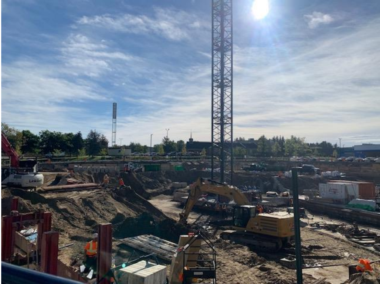
Figure 5: Existing Site Conditions at 1295 Bleams Road on September 26, 2024.
