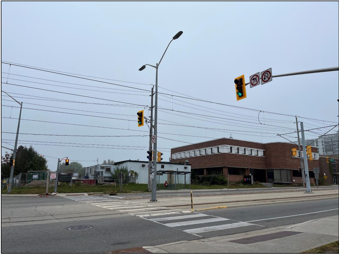
Figure 2 – View of Subject Lands (Intersection of King Street West and Pine Street)
